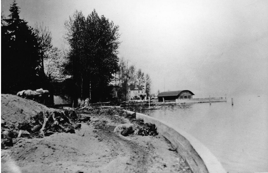
Construction of embankment at Denny-Blaine Park, view looking north – 1903 Seattle Municipal Archives - #17250
