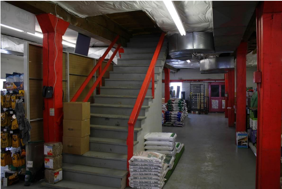
20 of 23. Rear stairwell on the interior of the Kennewick Fruit & Produce Co. Building. Camera facing southeast.
