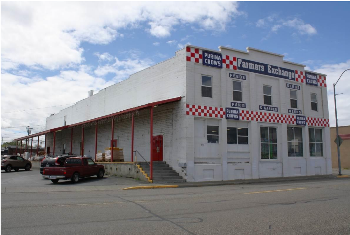
3 of 23. Northeast corner of the Kennewick Fruit & Produce Co. Building, showing north façade and east side. Camera facing southwest.
