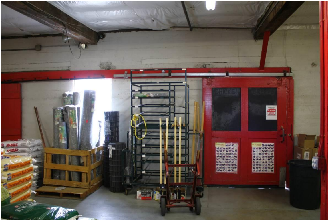
22 of 23. Interior view of the original wood door at the southwest corner of the Kennewick Fruit & Produce Co. Building. Camera facing south.
