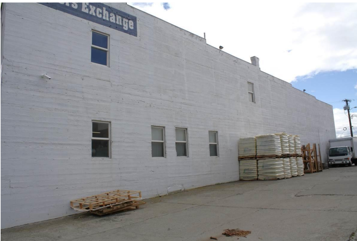
13 of 23. West side of the Kennewick Fruit & Produce Co. Building. Camera facing southeast.
