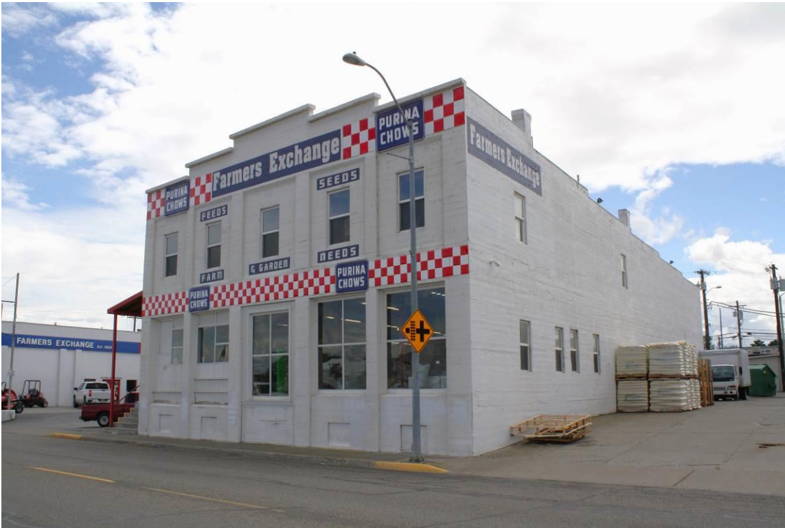
14 of 23. Northwest corner of the Kennewick Fruit & Produce Co. Building, showing north façade and west side. Camera facing southeast.
