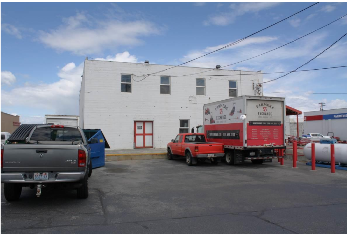
9 of 23. Rear, south end of the Kennewick Fruit & Produce Co. Building. Camera facing north.
