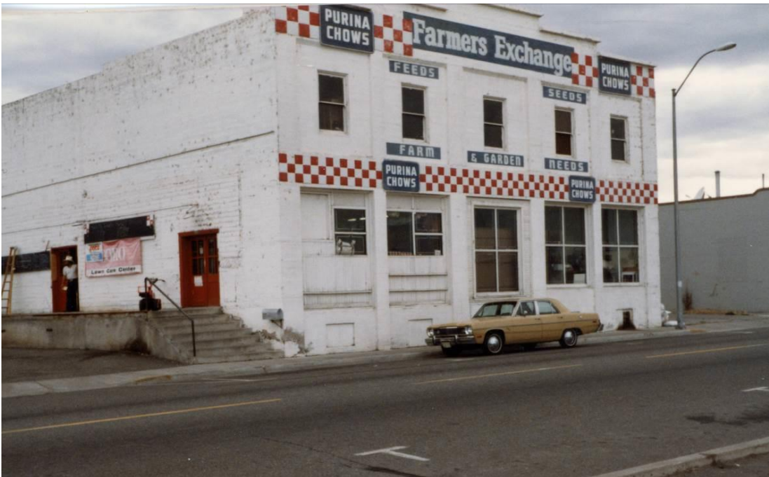
c.1980 photograph of the Farmers Exchange. Photograph courtesy of Chris Ingersoll.
