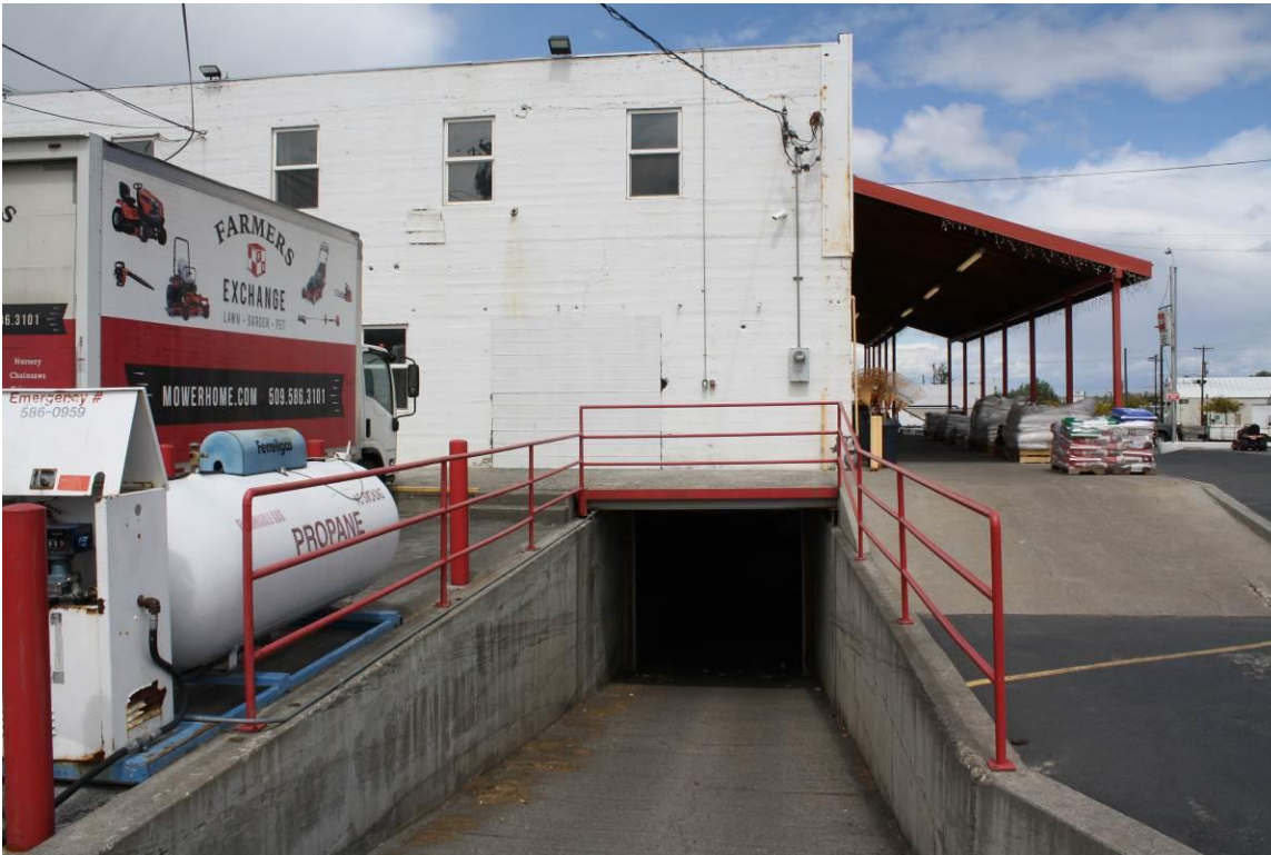
8 of 23. Loading ramp leading to the basement at the southeast corner of the Kennewick Fruit & Produce Co. Building. Camera facing north.
