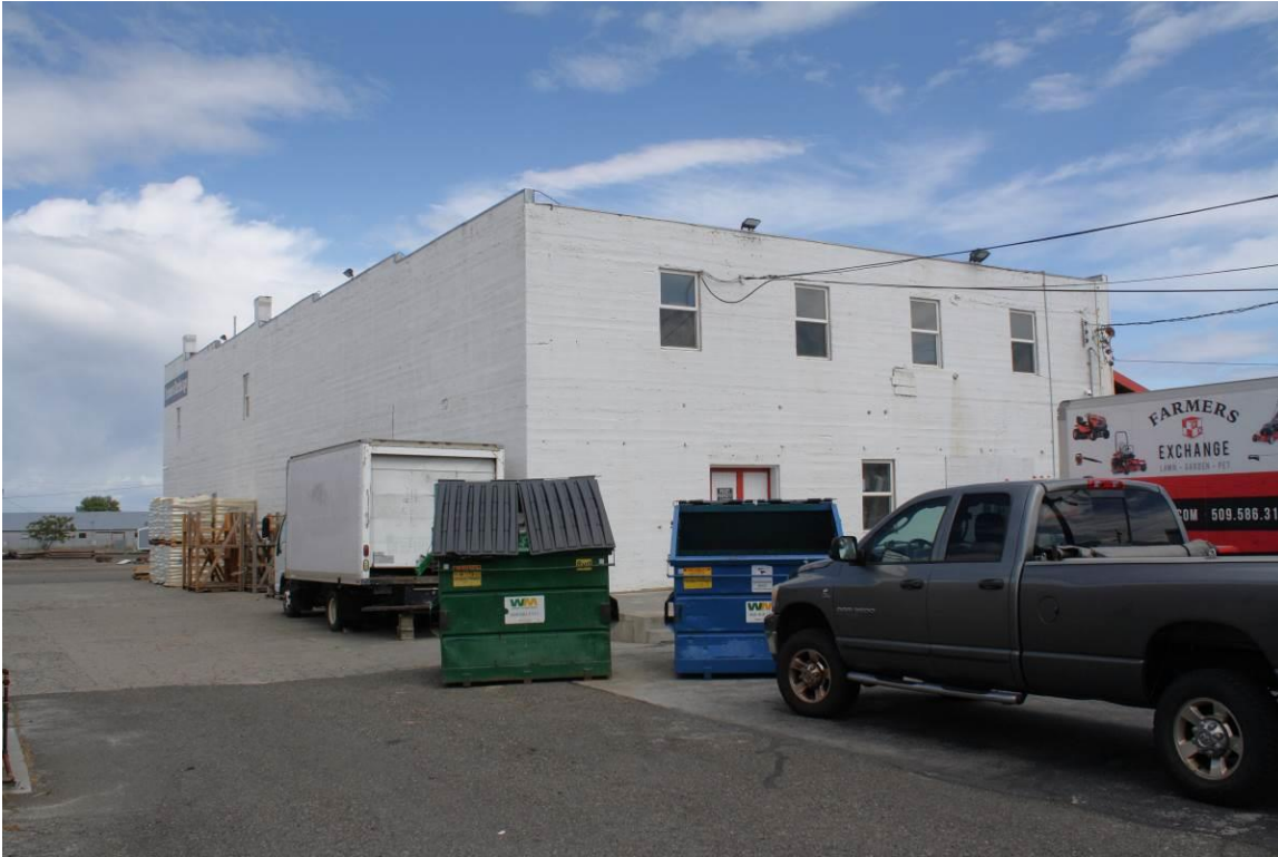
12 of 23. Southwest corner of the Kennewick Fruit & Produce Co. Building, showing south end and west side. Camera facing northeast.
