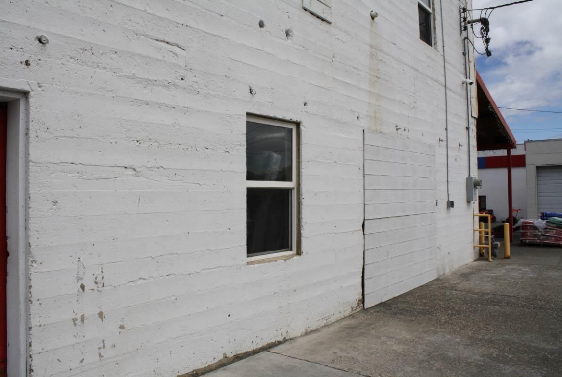
10 of 23. Detail view of replacement fenestration and door opening enclosed with wood boards on south side of the Kennewick Fruit & Produce Co. Building. Camera facing northwest.
