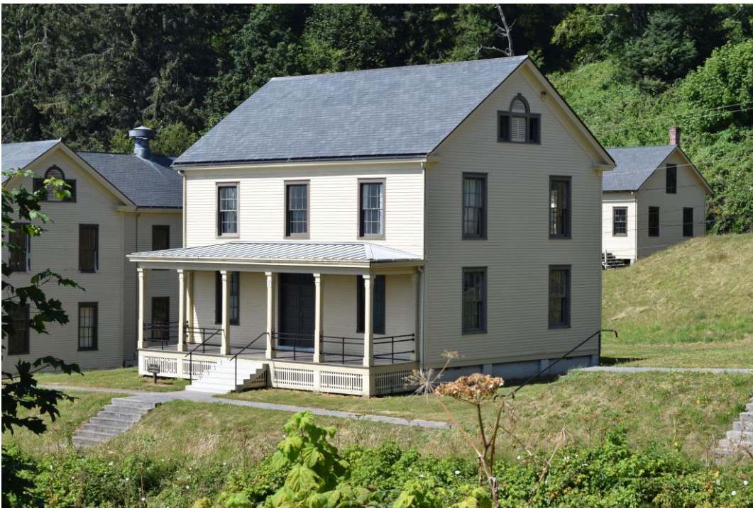
Photo 7. Administration Building (Site ID No. 3) looking north.
