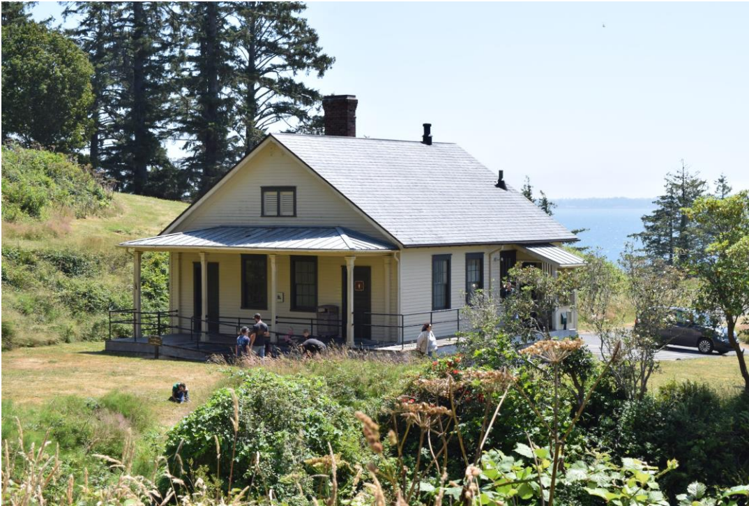
Photo 10. Guard House (Site ID No. 8) looking south.
