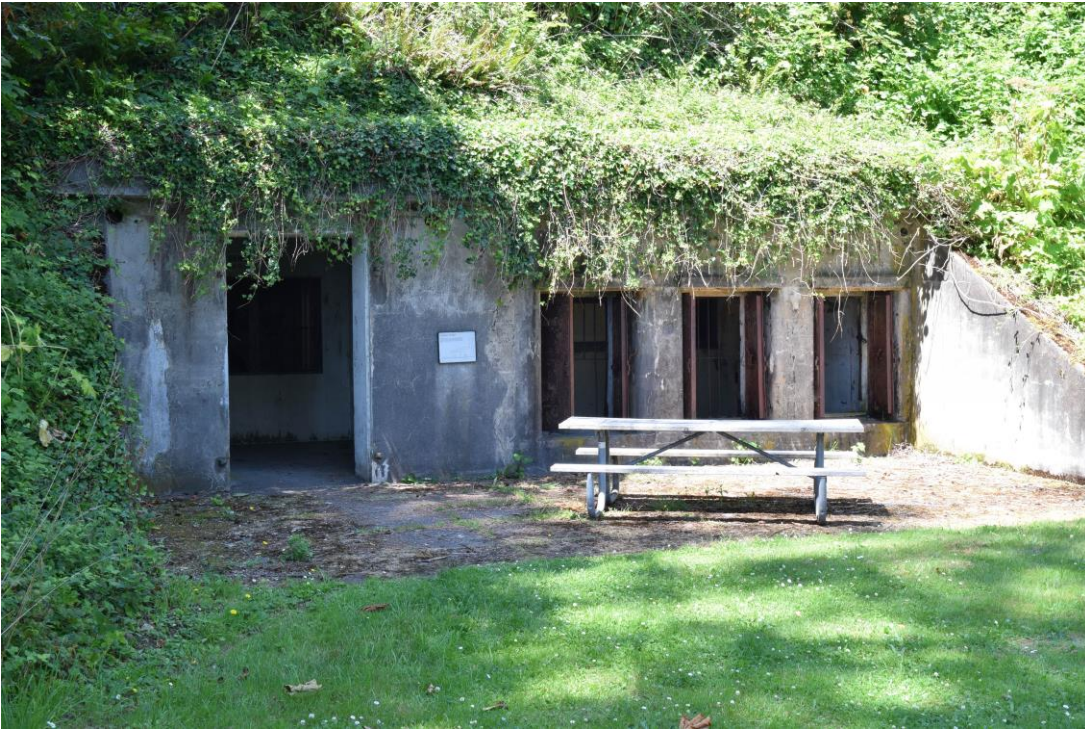
Photo 18. Looking northwest at Central Power Plant (Site ID No. 21)
