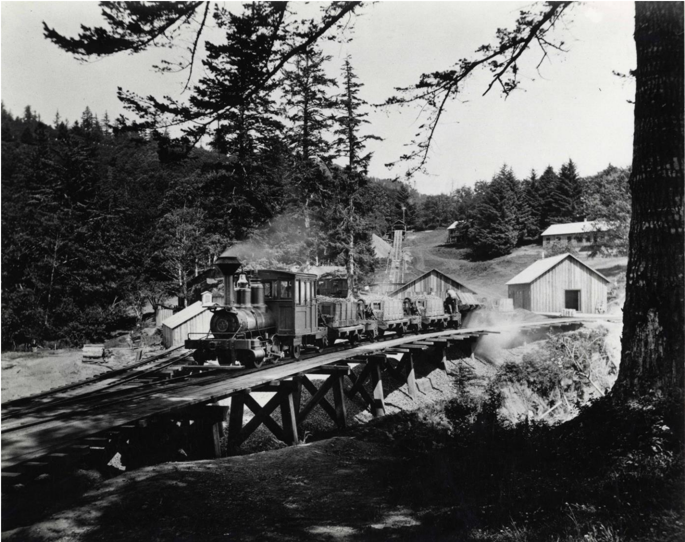
Construction in progress at Chinook Point in 1899. Shown are temporary buildings related to the construction of the fortifications; when no longer needed, the temporary buildings were removed to make room for the permanent buildings of the garrison. The tramway visible behind the rail cars leads to the site of the third emplacement of Battery Ord. Photo H39-203ft, Interpretive Collections, Washington State Parks and Recreation Commission.
