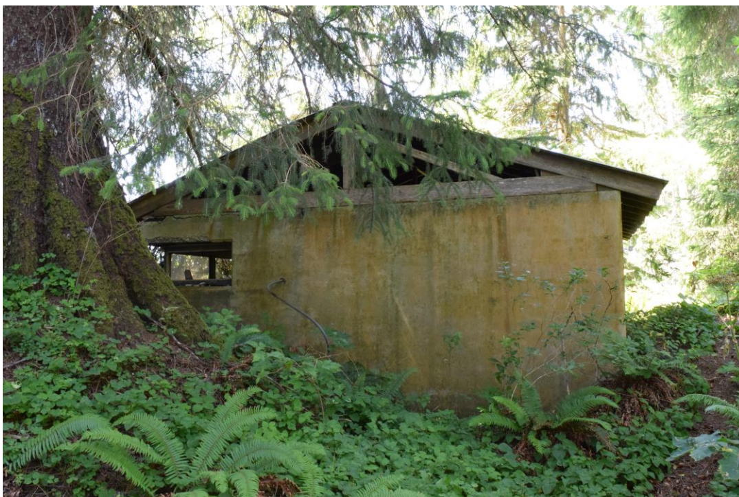
Photo 21. Looking northwest at side of the upper story of the Mine Command Station (Site ID No. 30) with observation opening to the left.
