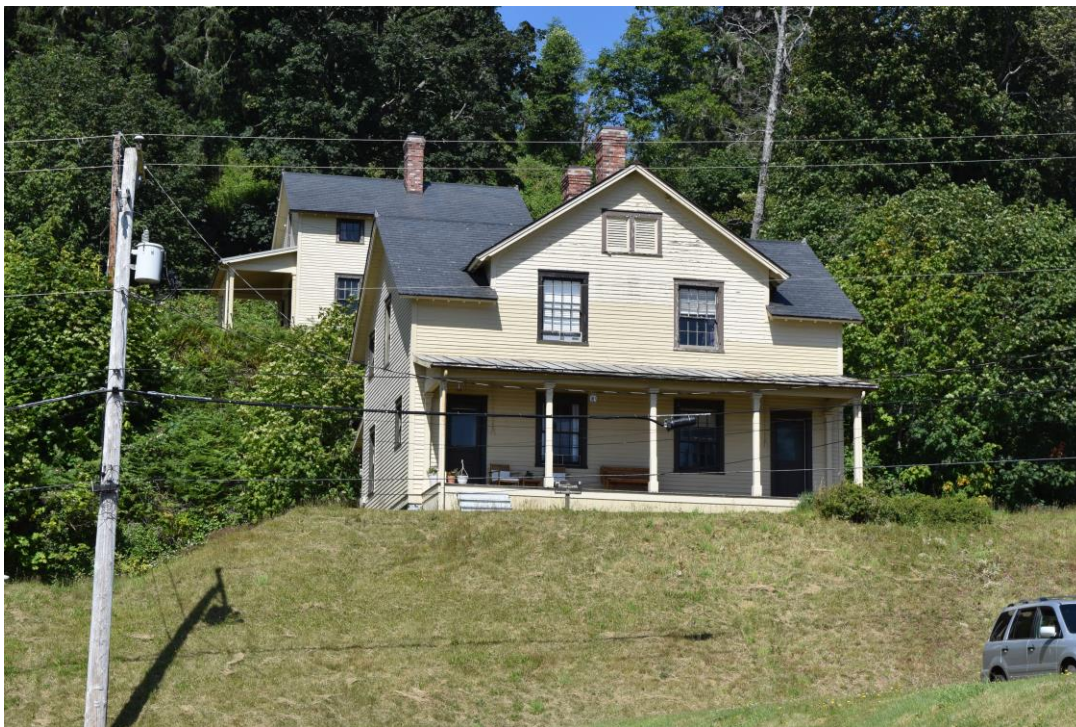
Photo 8. Non-commissioned Officers' Quarters (Site ID No. 4) looking north with Hospital Steward's Quarters (Site ID No. 5) partially visible to the rear.
