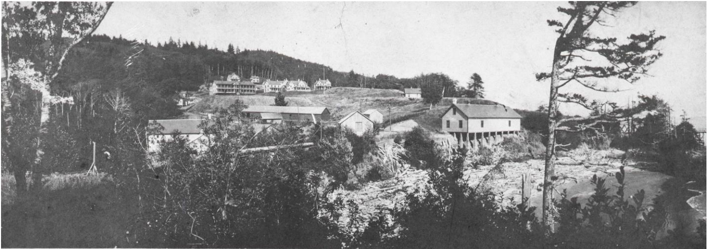
Fort Columbia prior to World War I looking to the east. To the left of center are a collection of temporary buildings remaining from the construction period. Prominent to the right of center is the Ordnance Storehouse (Site ID No. 11). Above and immediately to the left of the Ordnance Storehouse is the Guard House (Site ID No. 8) on its original location approximately between Batteries Crenshaw and Murphy. Photo 39-0-2016-1-H283, Interpretive Collections, Washington State Parks and Recreation Commission.
