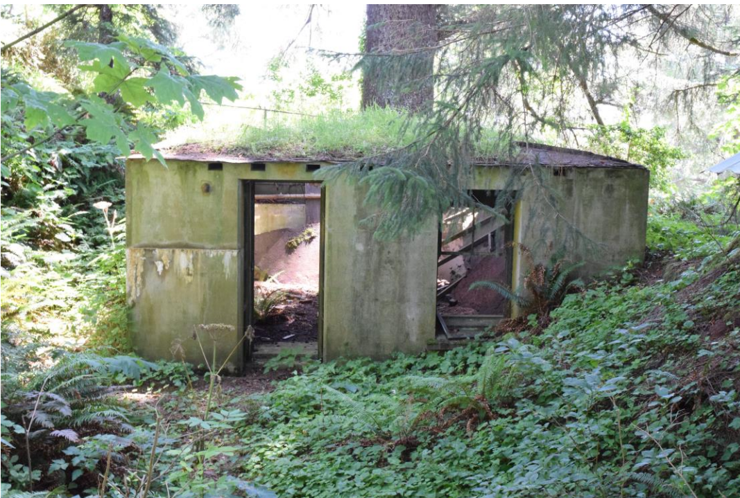
Photo 19. Looking southwest at rear entry to Battery Commander's Station Battery Ord (Site ID No. 29).
