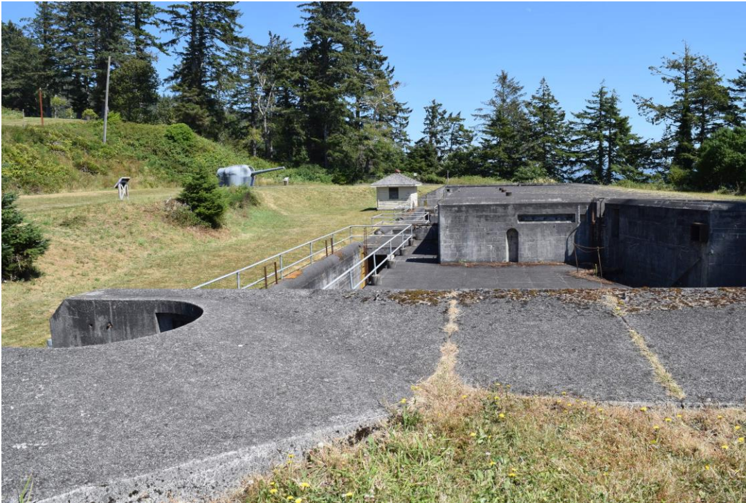
Photo 12. Looking east at Battery Murphy (Site ID No. 17) and its associated Latrine (Site ID No. 18). To the left is Gun No. 2 of Battery 246 (Site ID No. 22); most of the battery structure is hidden in the large mound behind the gun.
