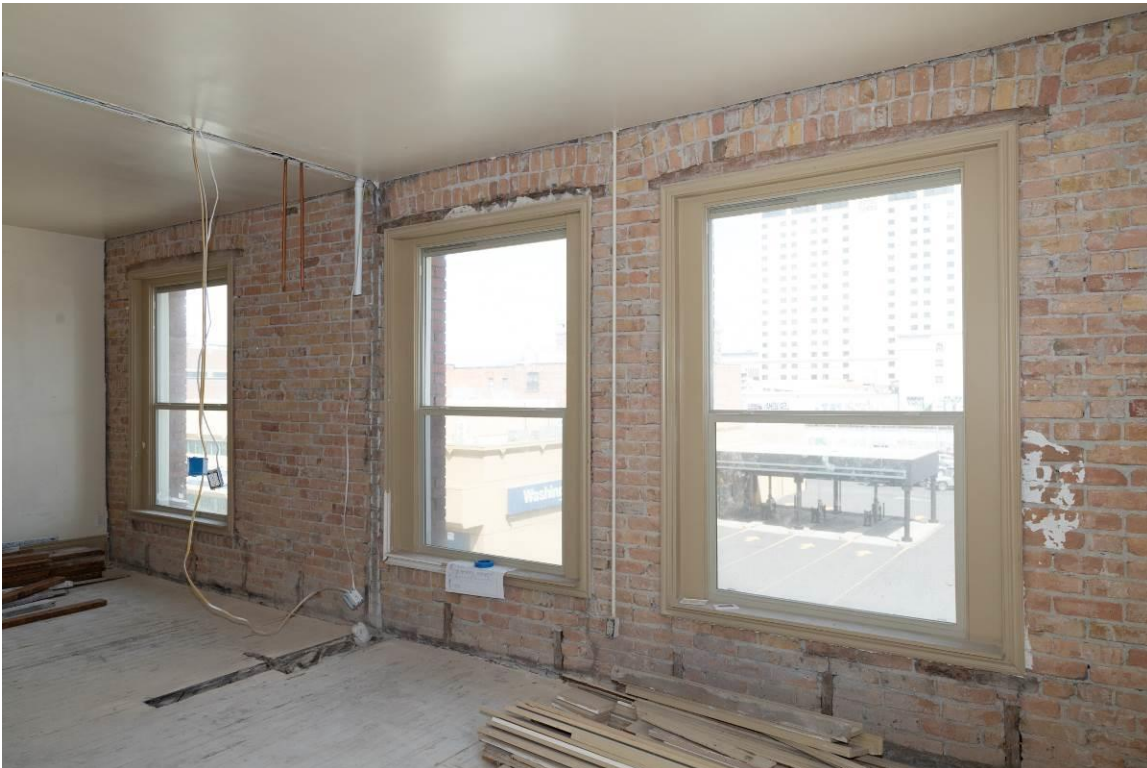
WA_Spokane County_Hotel Collins_0047. Third floor, northeast corner unit, looking northwest.
