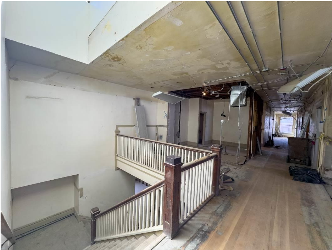
WA_Spokane County_Hotel Collins_0041. Third floor, central stairwell, looking southeast.
