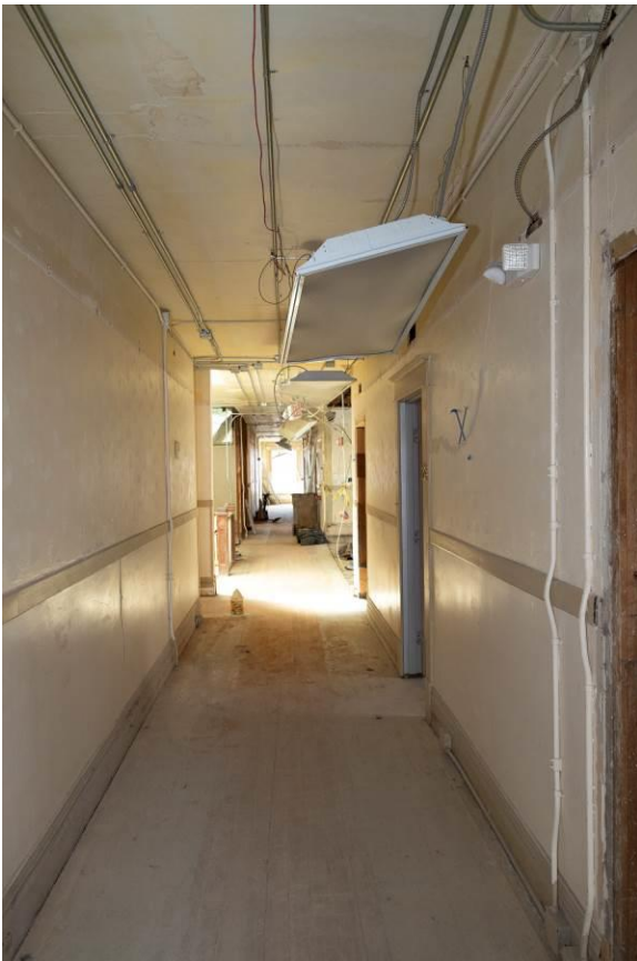
WA_Spokane County_Hotel Collins_0043. Third floor, main hallway, looking south.
