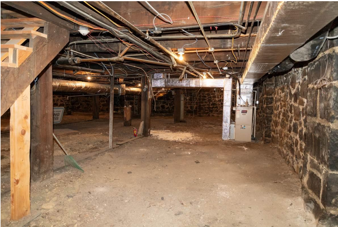
WA_Spokane County_Hotel Collins_0015. Basement, looking north.
