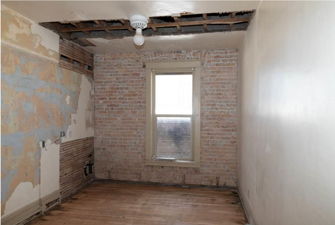
WA_Spokane County_Hotel Collins_0050. Third floor, west unit, looking west.
