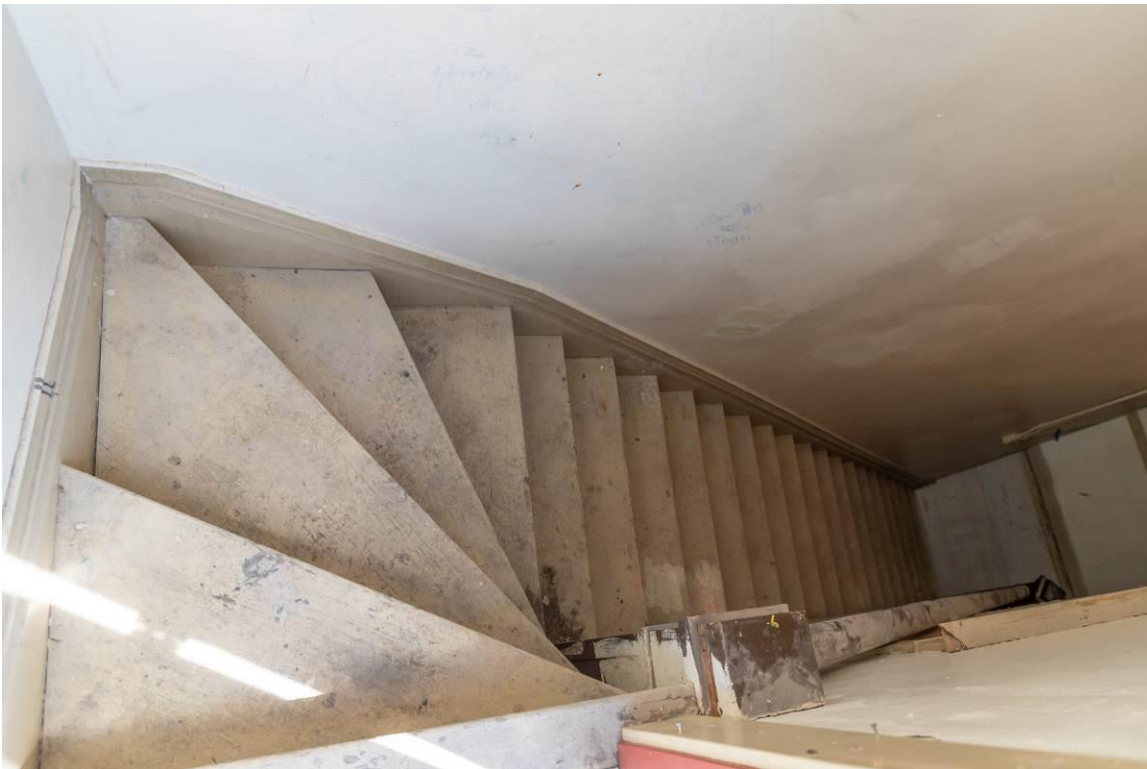
WA_Spokane County_Hotel Collins_0053. Roof, stairway down to the third floor.
