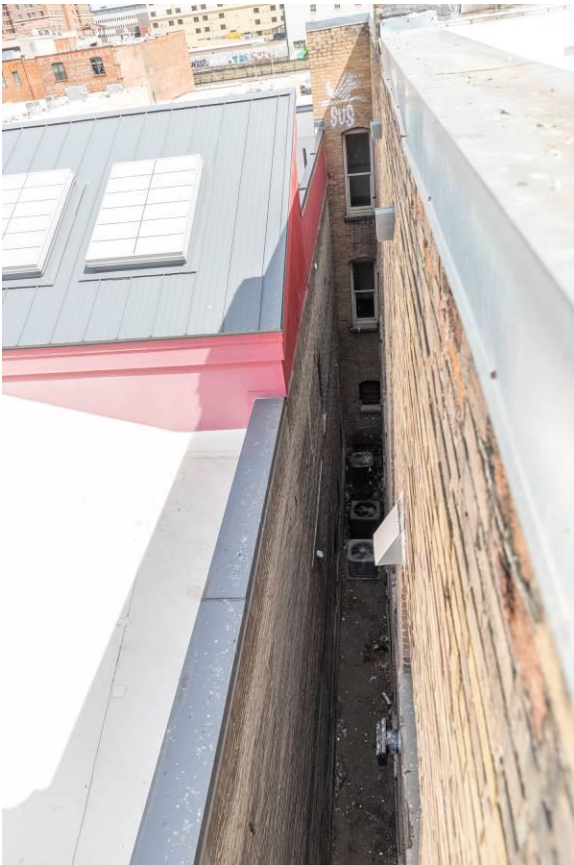
WA_Spokane County_Hotel Collins_0011. Roof, light well, looking north.
