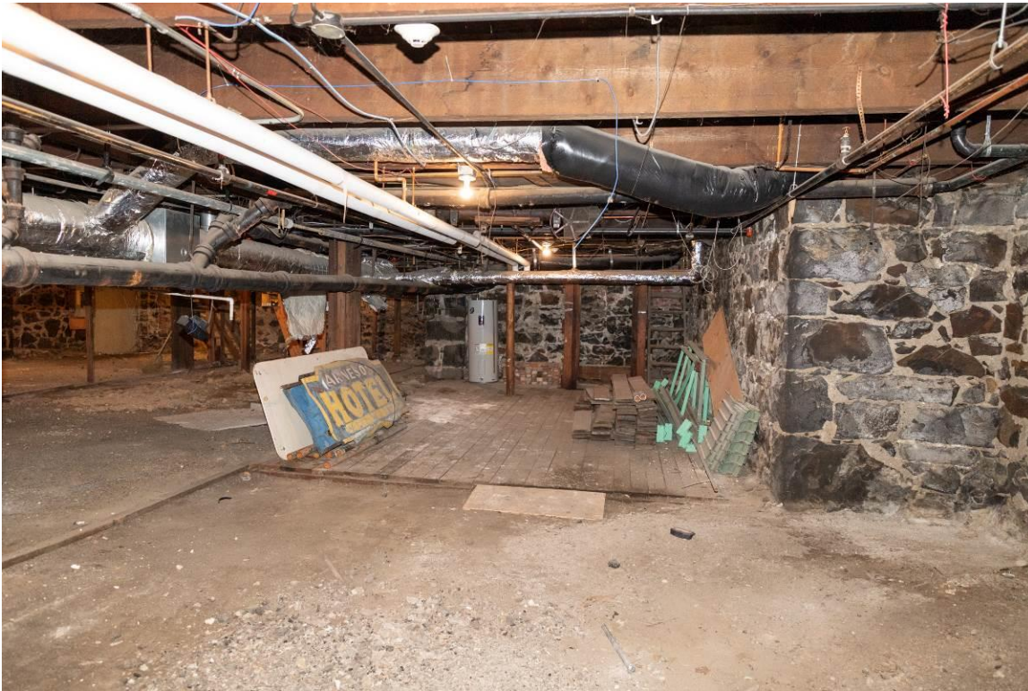
WA_Spokane County_Hotel Collins_0016. Basement, looking south.
