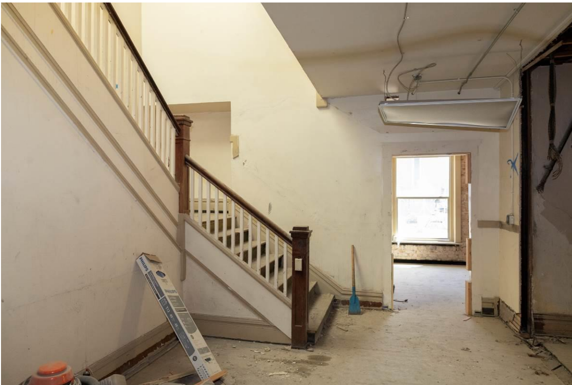
WA_Spokane County_Hotel Collins_0023. Second floor, central stairwell, looking east.
