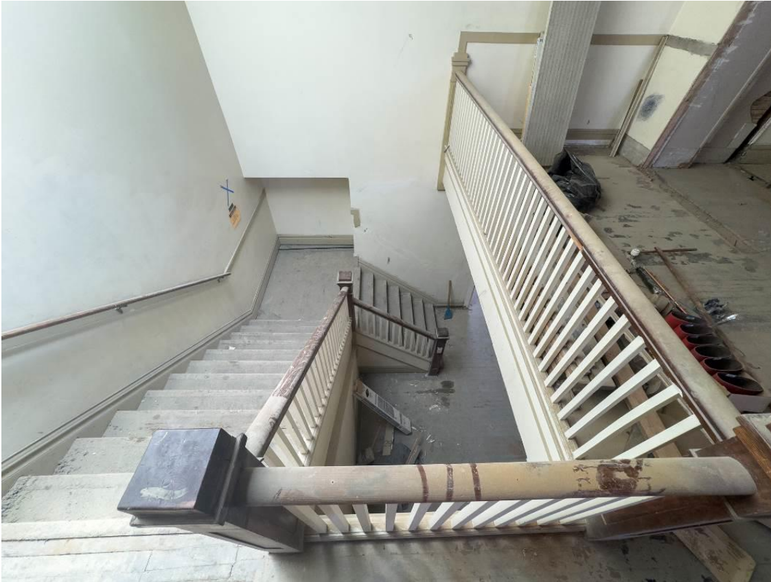
WA_Spokane County_Hotel Collins_0040. Third floor, central stairwell, looking east and down.
