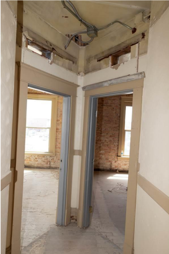
WA_Spokane County_Hotel Collins_0046. Third floor, east branch hallway, looking east.
