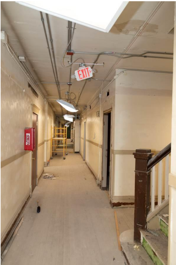
WA_Spokane County_Hotel Collins_0027. Second floor, main hallway, looking south.
