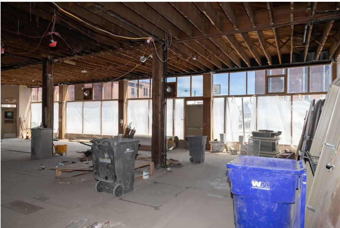
WA_Spokane County_Hotel Collins_0019. First floor, looking north east towards the storefronts.
