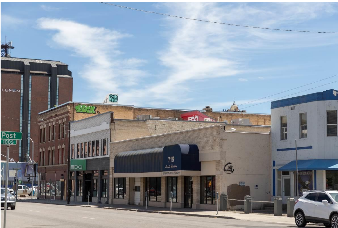
WA_Spokane County_Hotel Collins_0005. Exterior, west facade.
