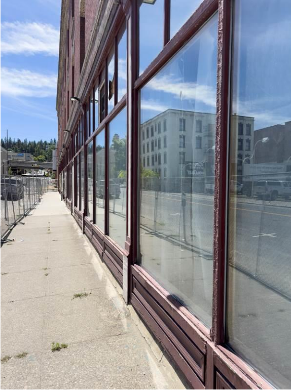
WA_Spokane County_Hotel Collins_0006. Exterior, storefronts along South Wall Street, looking south.
