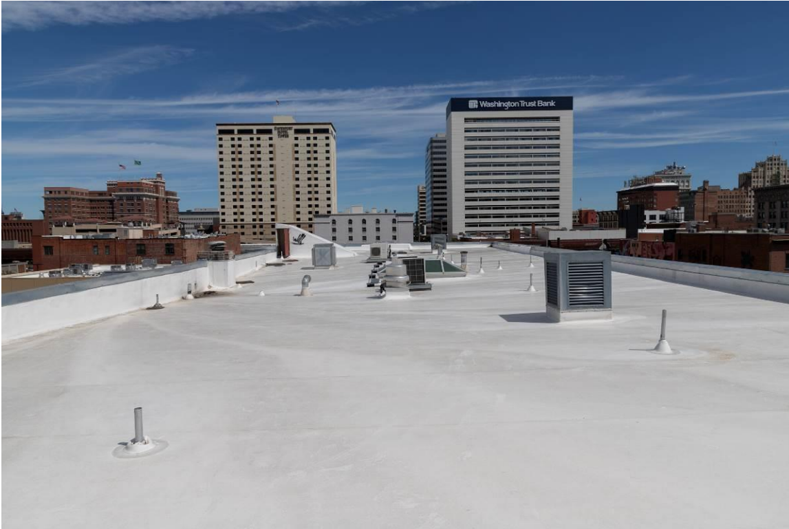
WA_Spokane County_Hotel Collins_0010. Roof, looking north.
