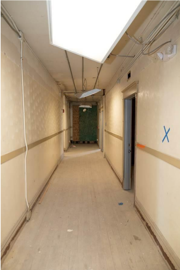
WA_Spokane County_Hotel Collins_0028. Second floor, main hallway, looking south.
