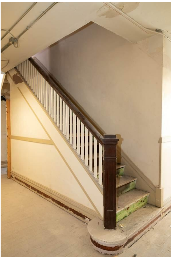
WA_Spokane County_Hotel Collins_0039. Second floor, northwest stairway, looking northwest.
