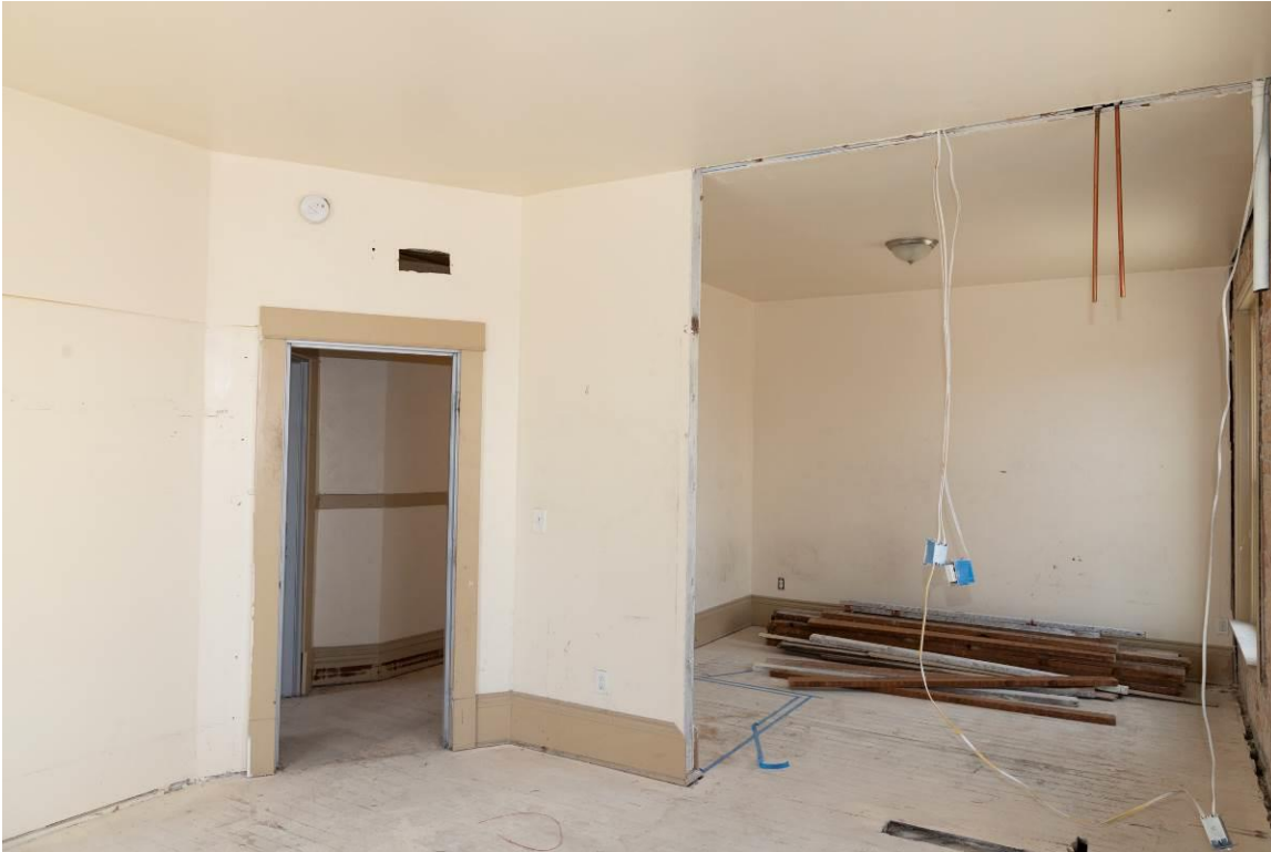
WA_Spokane County_Hotel Collins_0048. Third floor, northeast corner unit, looking southwest.
