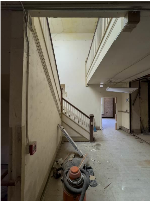
WA_Spokane County_Hotel Collins_0025. Second floor, central stairwell, looking east.
