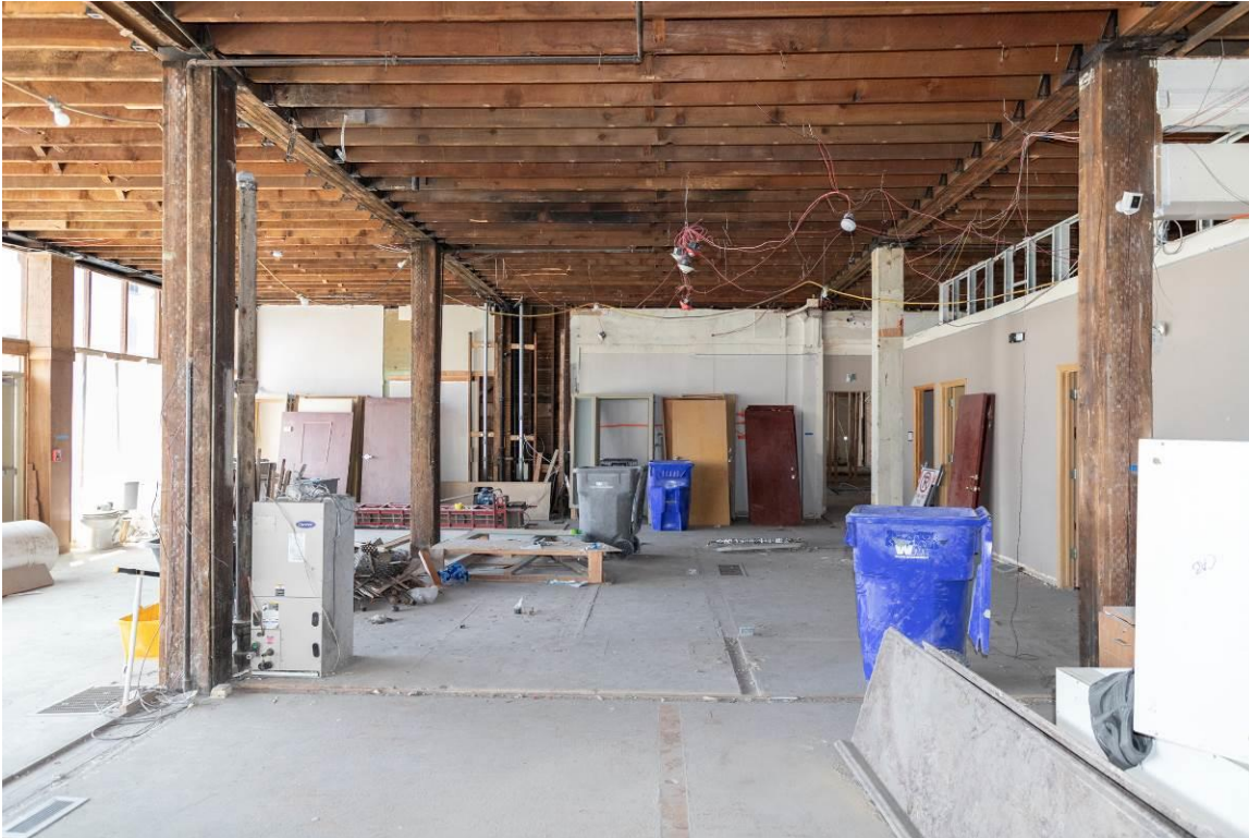
WA_Spokane County_Hotel Collins_0020. First floor, looking south.
