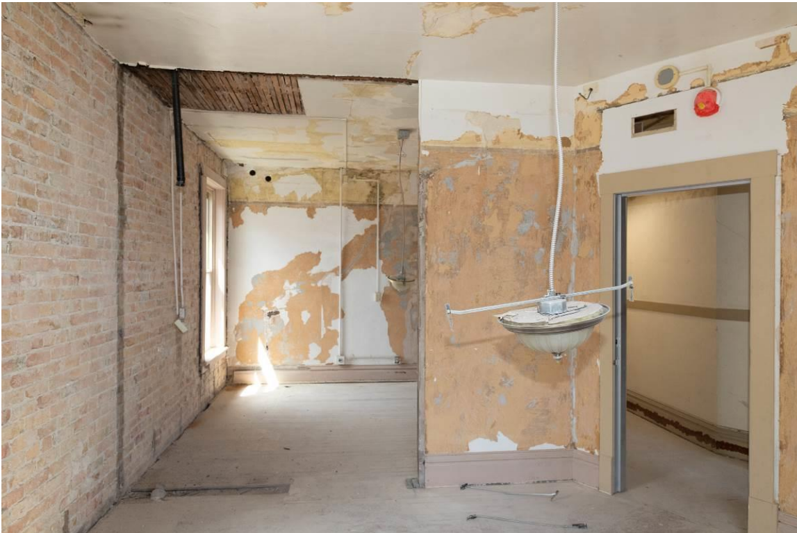
WA_Spokane County_Hotel Collins_0033. Second floor, southeast corner unit, looking west.
