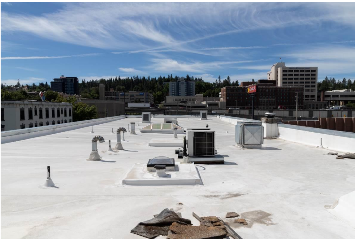
WA_Spokane County_Hotel Collins_0009. Roof, looking south.
