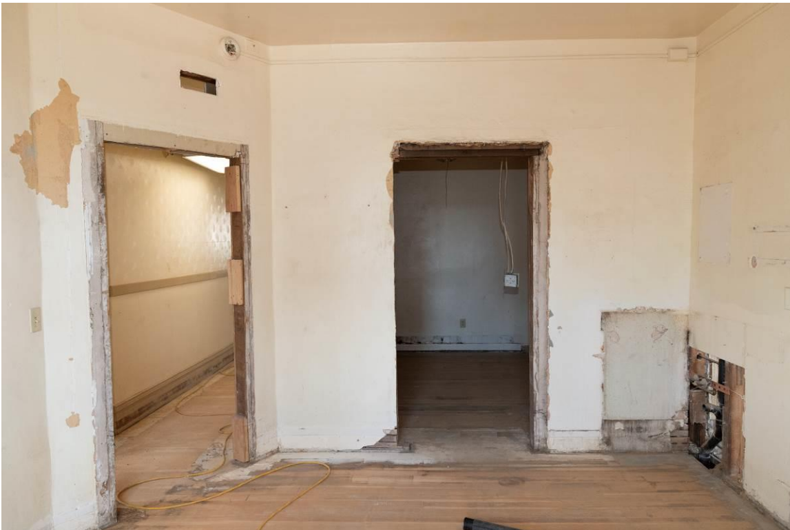
WA_Spokane County_Hotel Collins_0049. Third floor, east unit, looking west.
