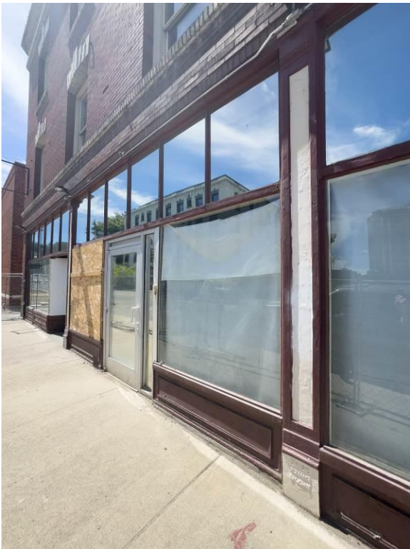
WA_Spokane County_Hotel Collins_0007. Exterior, east facade storefronts, looking south.
