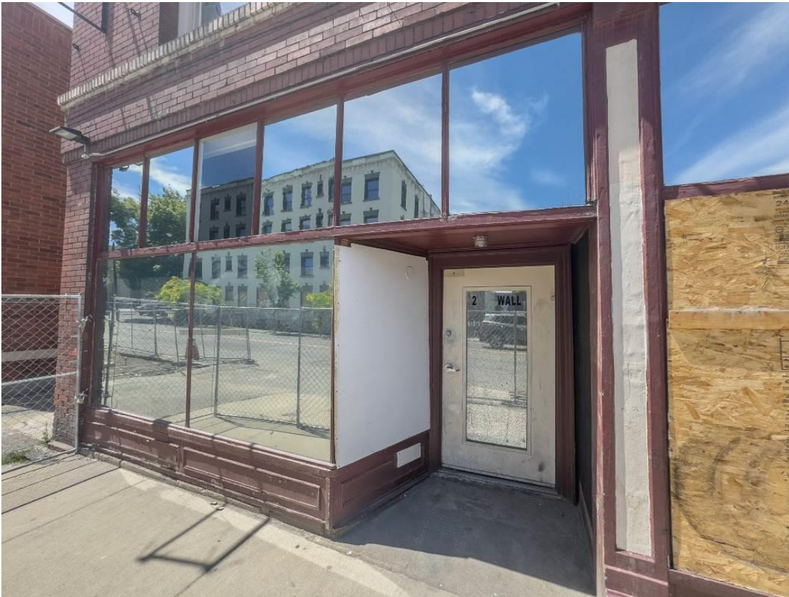
WA_Spokane County_Hotel Collins_0008. Exterior, 212 South Wall Street entrance.
