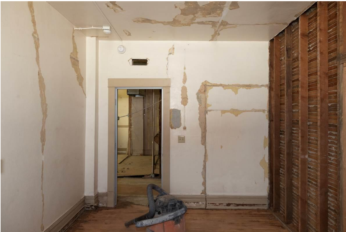
WA_Spokane County_Hotel Collins_0051. Third floor, west unit, looking east.
