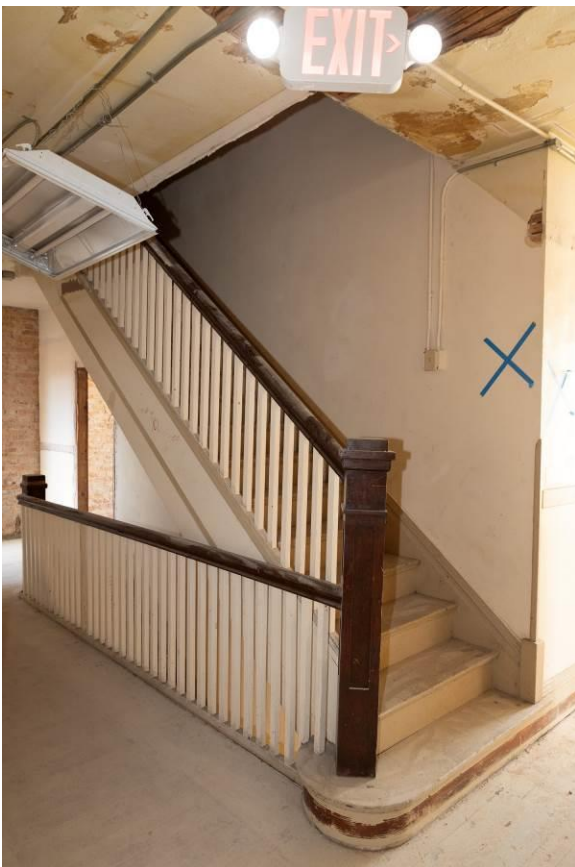
WA_Spokane County_Hotel Collins_0045. Third floor, northwest stairway, looking northwest.
