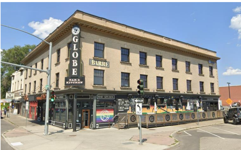
Fig. 14. Globe Hotel (1908), 204 N Division Street, Spokane. Individually listed to the NRHP under the SRO MPD and as a contributing property in the East Downtown Historic District. Courtesy of Google StreetView.
