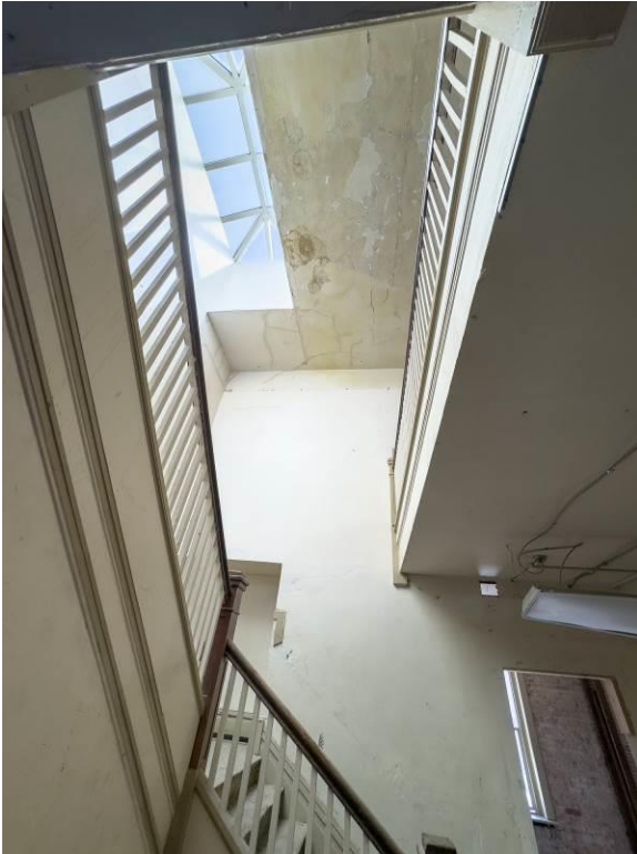
WA_Spokane County_Hotel Collins_0026. Second floor, central stairwell, looking east and up.
