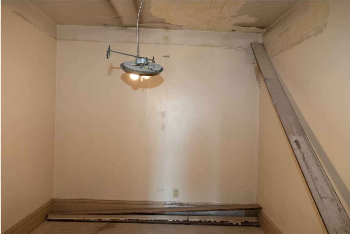
WA_Spokane County_Hotel Collins_0036. Second floor, east side unit, looking west.
