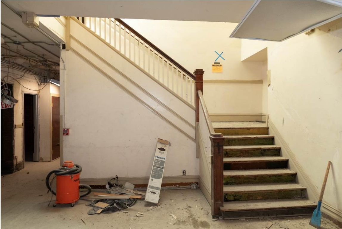
WA_Spokane County_Hotel Collins_0024. Second floor, central stairwell, looking north.
