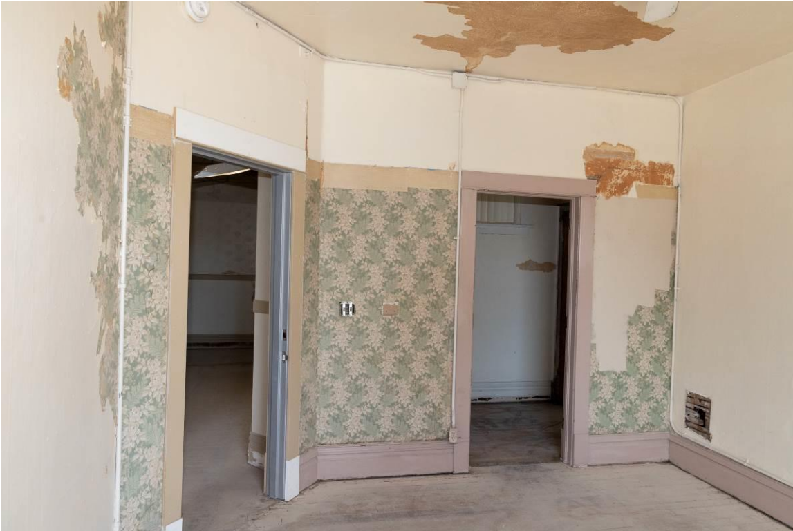
WA_Spokane County_Hotel Collins_0052. Third floor east unit, looking west.
