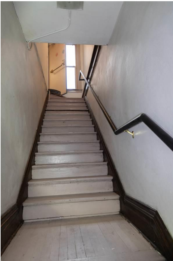
WA_Spokane County_Hotel Collins_0037. Second floor, northwest stairwell, looking up from the intermediate landing.
