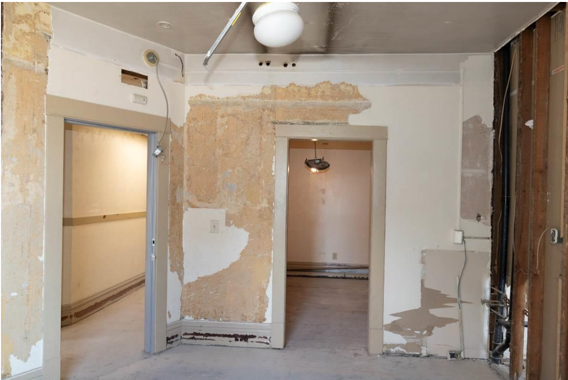
WA_Spokane County_Hotel Collins_0035. Second floor, east side unit, looking west.
