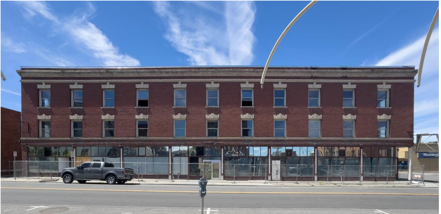
WA_Spokane County_Hotel Collins_0003. Exterior, front east facade, South Wall Street.
