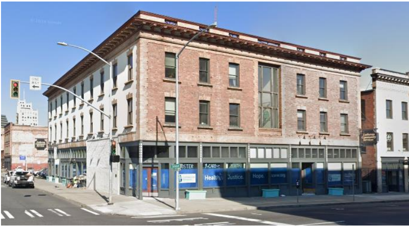
Fig. 13. Alger-Bristol Hotel (1904), 210 W Sprague Avenue, Spokane. Individually listed to the NRHP under the SRO MPD and as a contributing property in the East Downtown Historic District. Courtesy of Google StreetView.
