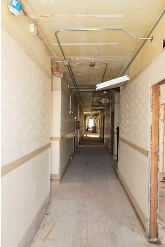
WA_Spokane County_Hotel Collins_0044. Third floor, main hallway, looking south.
