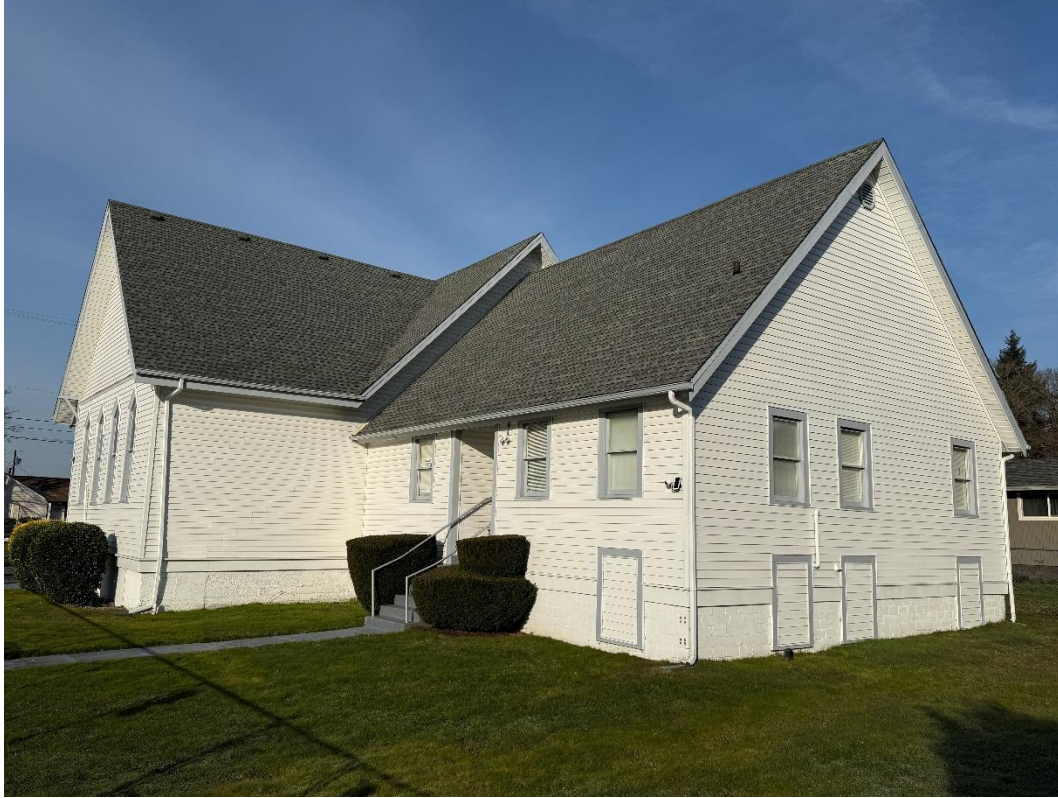
View of east side of building showing 1944 annex.
