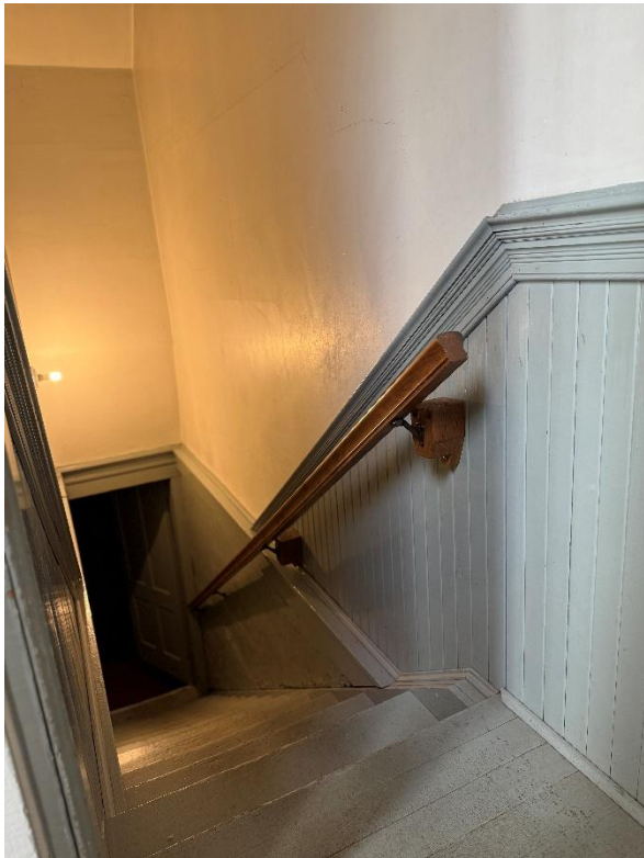
Detail of basement stairs.
