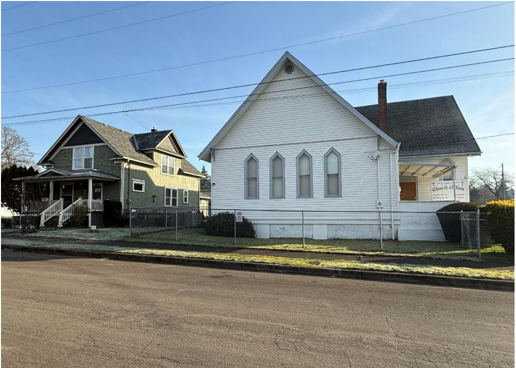
View of west facade of sanctuary showing 1910 parsonage (far left).
