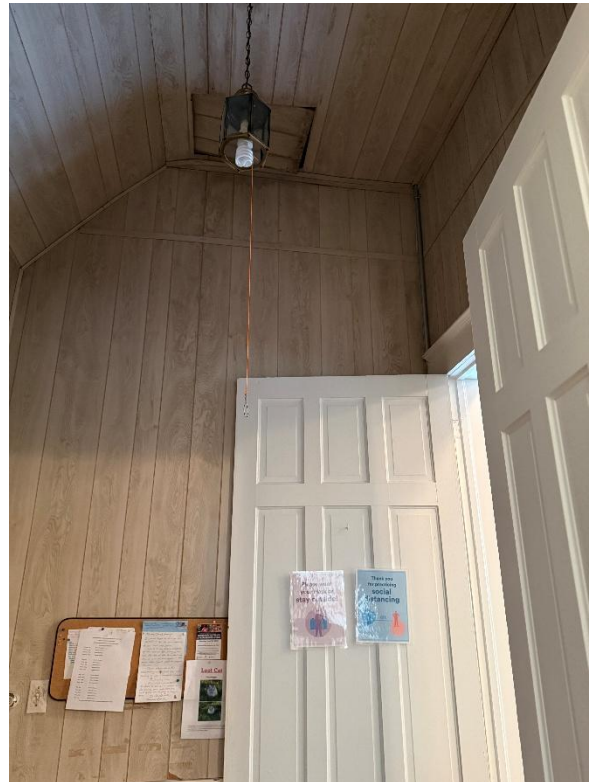
Detail of former bell tower entry vestibule.
