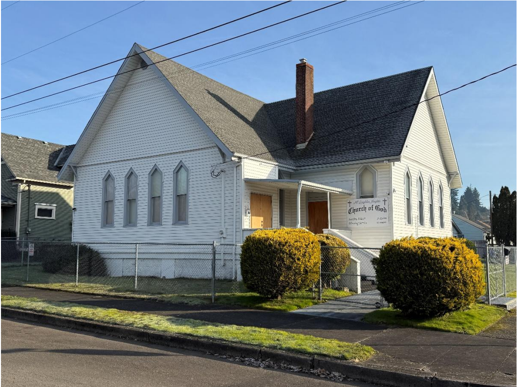
View of southwest corner of sanctuary.
