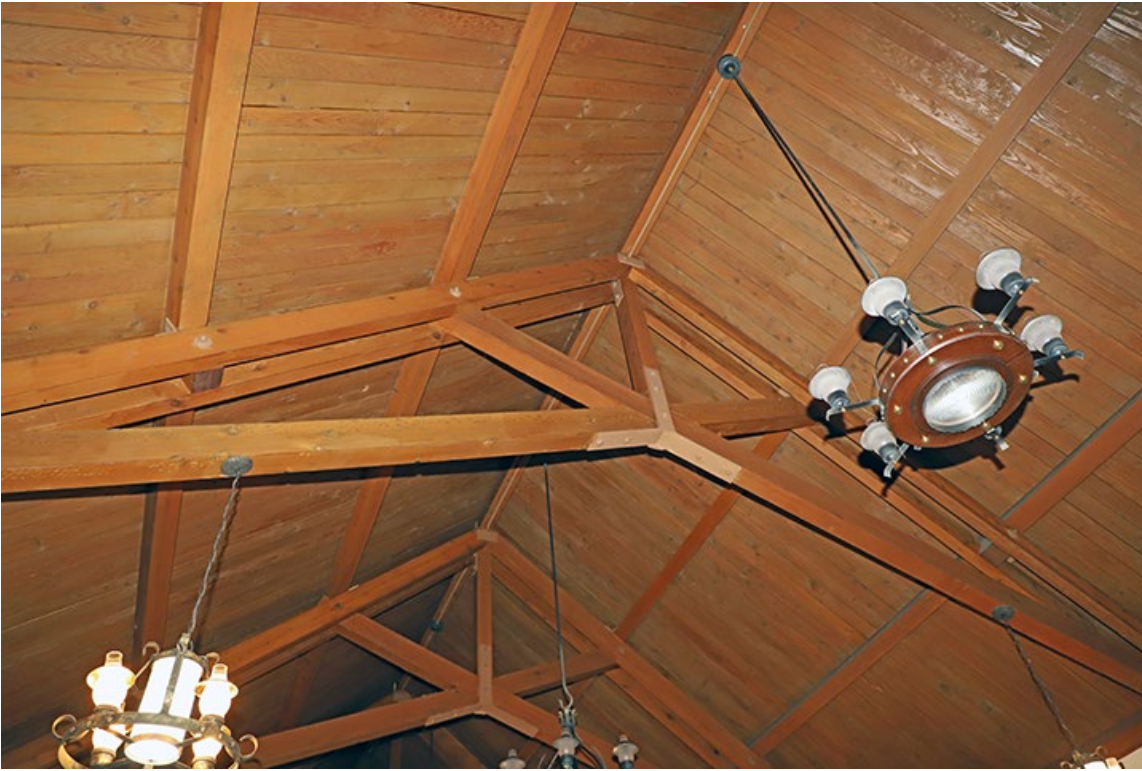
WA_KingCounty_NavalHospitalChapel_0043. Scissor Truss and light fixture detail.
