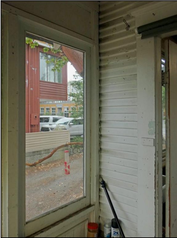
Photo 6 of 11. Enclosed rear porch window; view toward the northwest.
