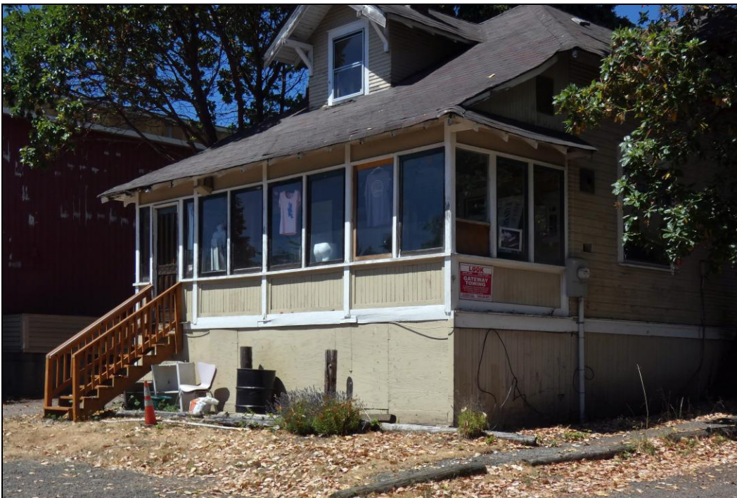
Photo 3 of 11. South face of the house with the enclosed rear porch and roof alterations.
