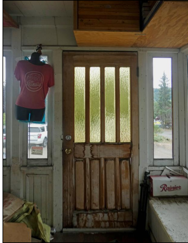
Photo 7 of 11. Exit door of enclosed rear porch; faces toward the south.
