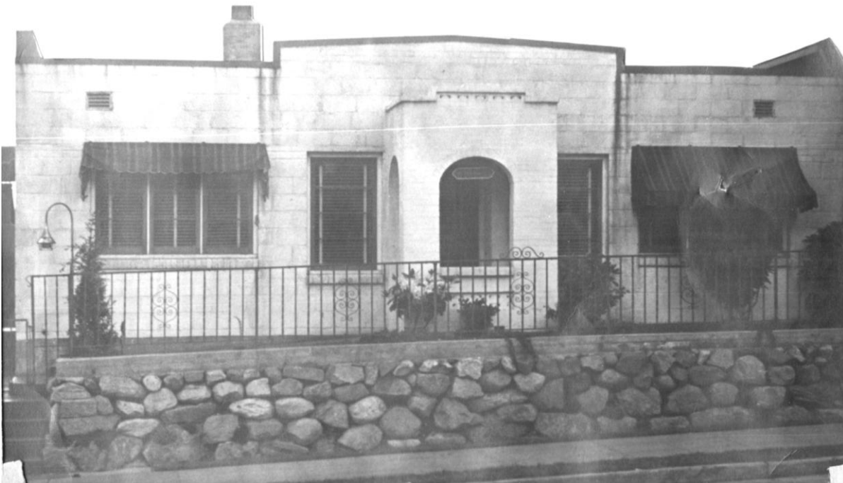
Eng House primary (east) elevation of the house, ca. 1940s.
