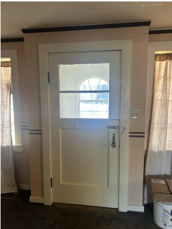
10 of 16: Detail of front door interior, camera facing east.
