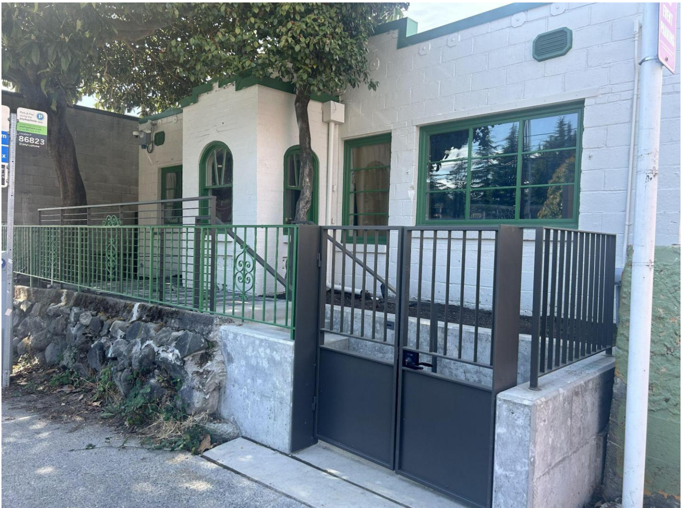
1 of 16: Primary (east) elevation of the house, camera facing southwest.
