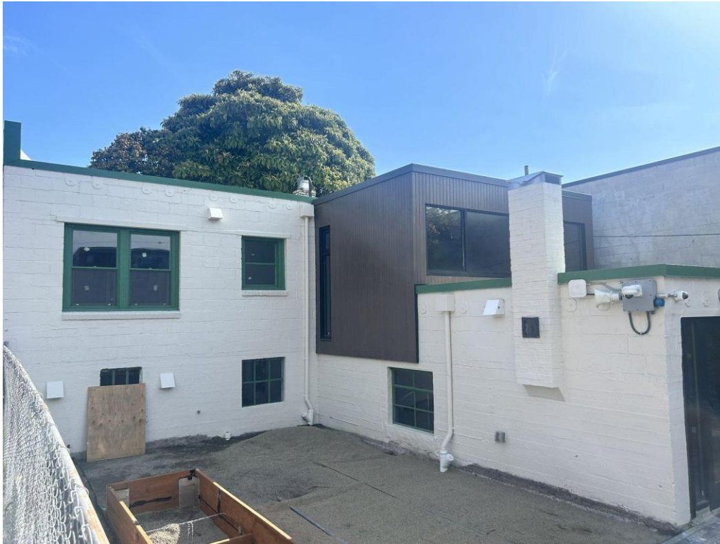
4 of 16: West elevation of the house and garage, camera facing southeast.
