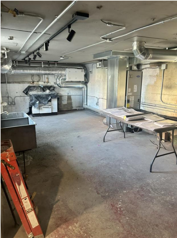
12 of 16: Basement space, camera facing northeast.
