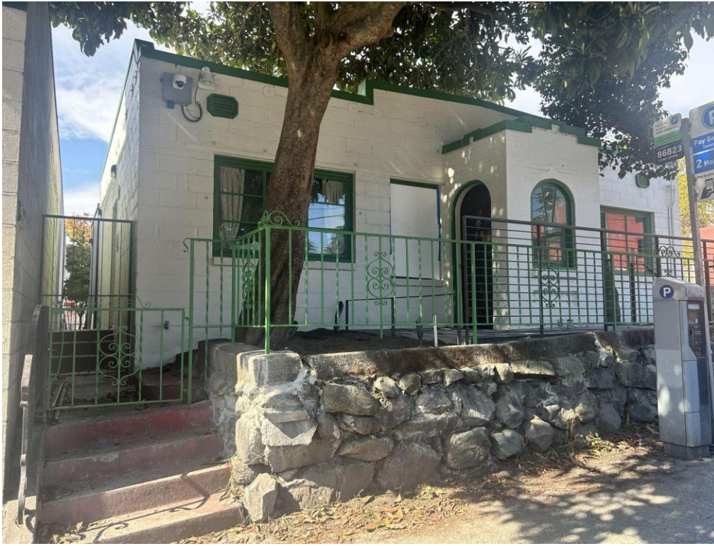
2 of 16: Primary elevation of the house, camera facing northwest.
