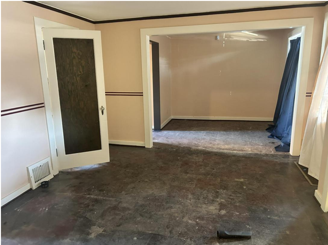
6 of 16: Interior of the house, looking at the north half of the living room and into the bedroom. The opening has been enlarged for future interpretive use by the Wing Luke Museum. Camera facing north.
