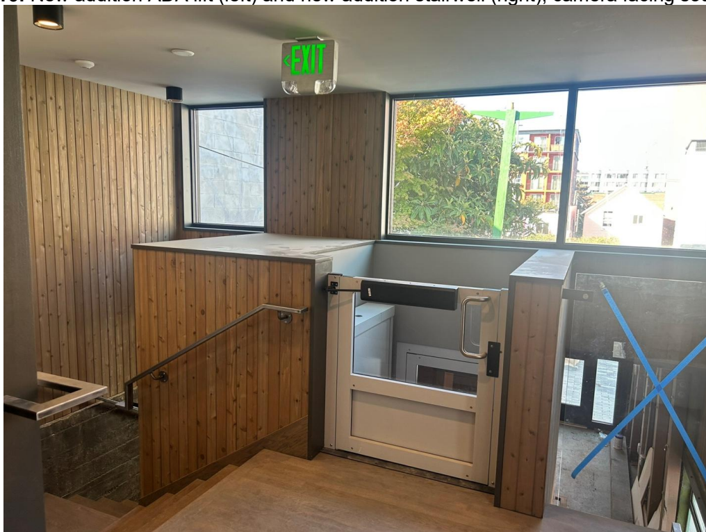
16 of 16: Landing area for new addition, camera facing west.
