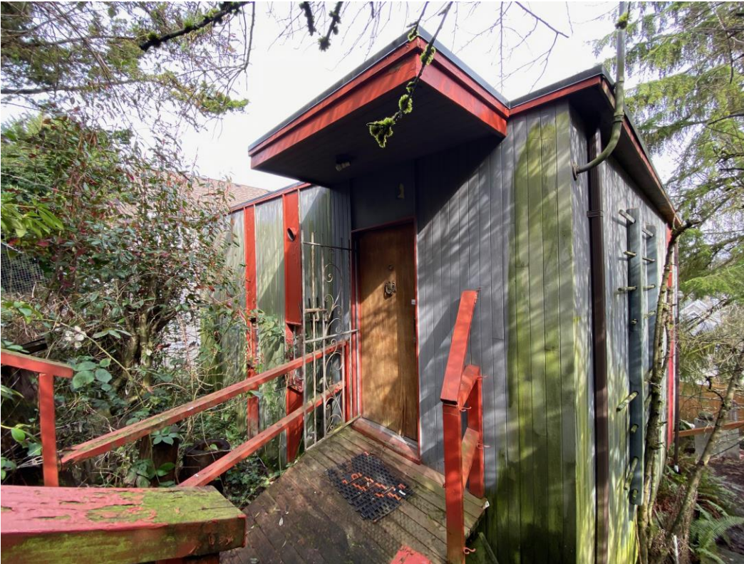
16 of 31 Main façade of Washington House – Detail of front entry porch.
