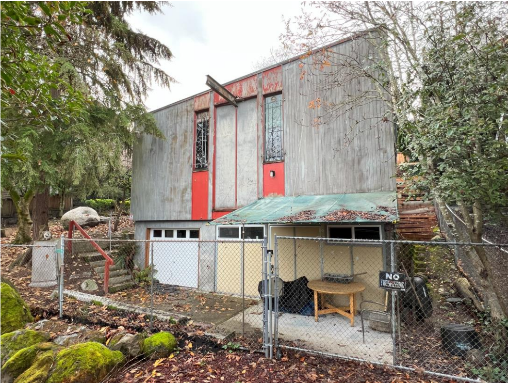
18 of 31 Studio east façade showing access from alleyway.
