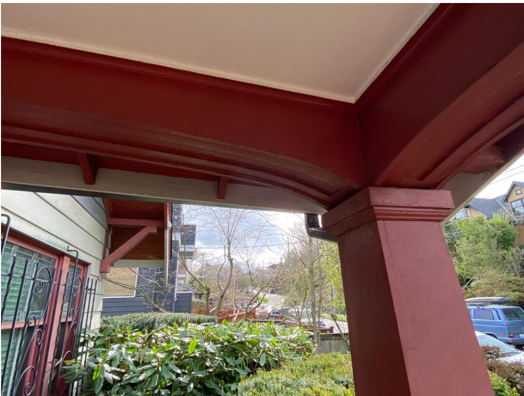
3 of 31 Main façade of Washington House – Detail of front entry porch corner.
