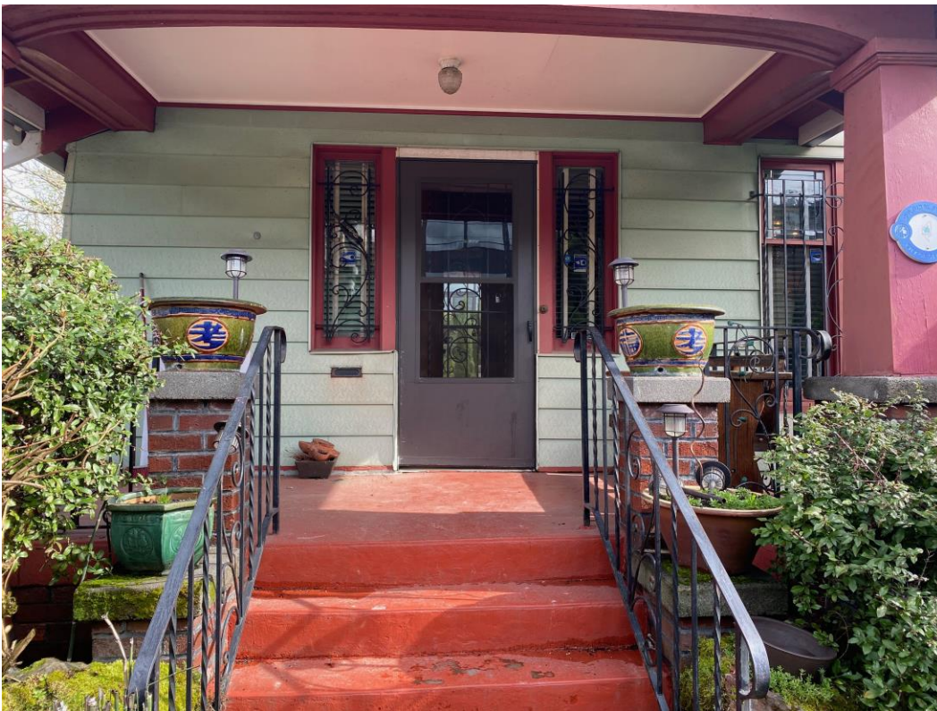
2 of 31 Main façade of Washington House – Detail of front entry porch.
