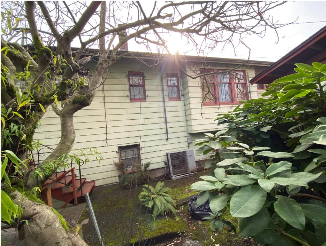
4 of 31 North façade of Washington House.
