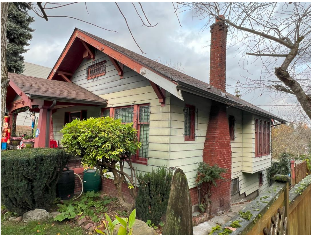
7 of 31 Southwest corner of Washington House – View of south facade.
