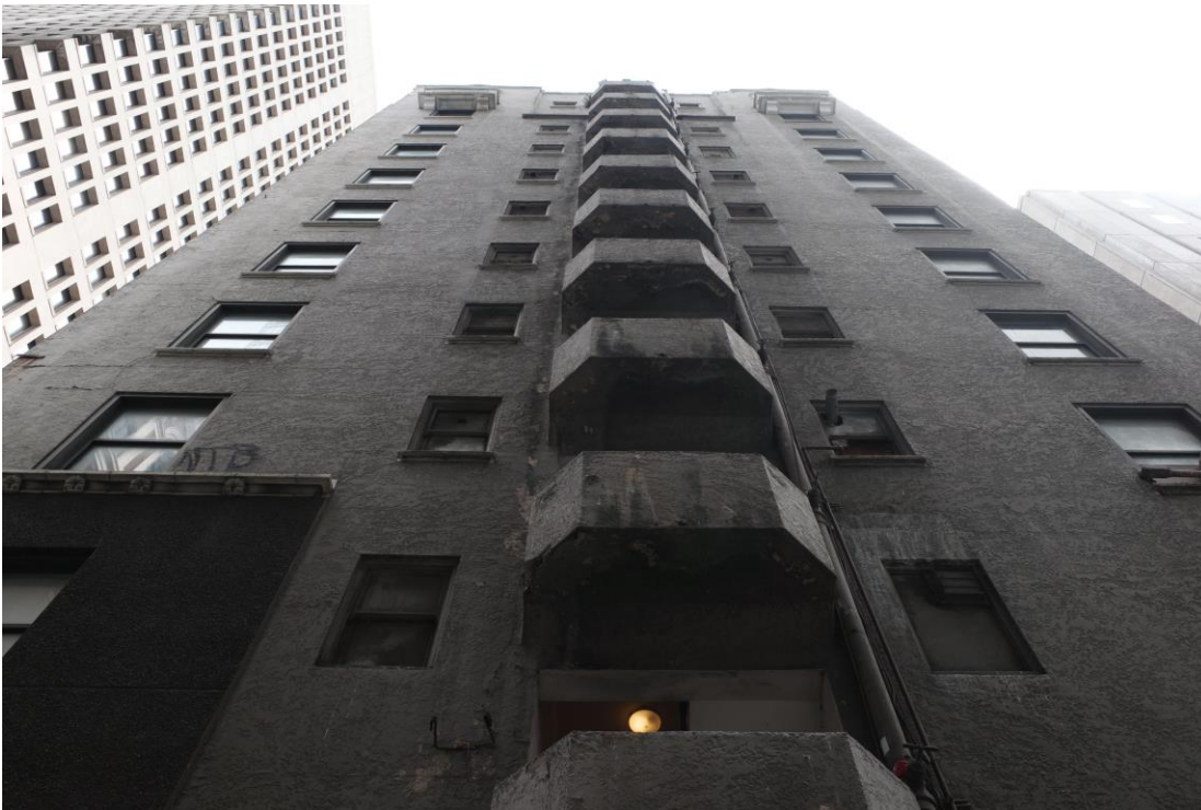
0007. Looking upward at the west façade showing cast concrete exit stairs above the alley. Weinstein AU photographer, June 16, 2021.
