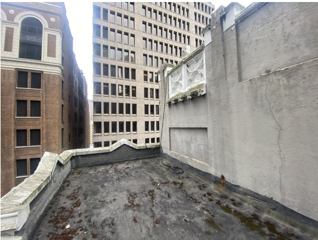
0008. Northwest corner on the on the tenth floor roof deck showing a decorative terra cotta panel and parapet caps. Weinstein AU photographer, May 21, 2021.
