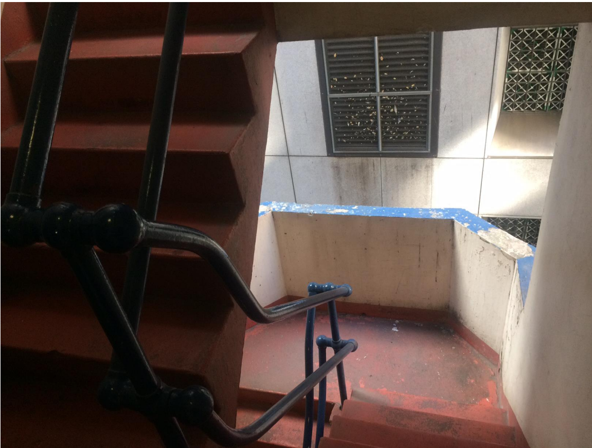
0018. Looking west at the painted concrete exterior exit stairs with low surrounding wall and pipe railings. Susan Boyle photographer, September 2, 2021.
