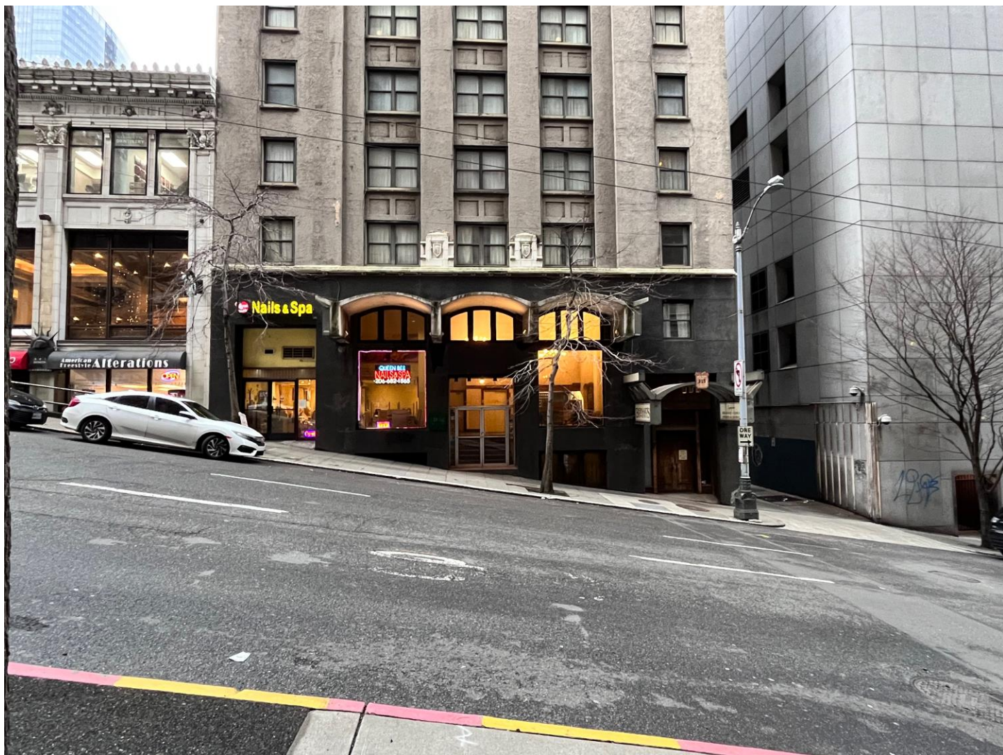
0009. Looking south at the lower level north façade showing the arrangement of entries, and non-original cladding and canopies, along with the terra cotta trim band below the second floor windows and cast panels below the paired windows in the central bays above. Susan Boyle photographer, February 3, 2022.
