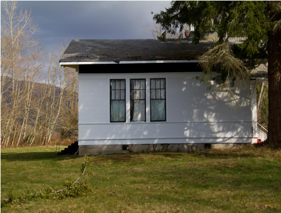
4 of 14. Side (west) elevation facing east of 1916 schoolhouse. Photo labeled as WA_SkagitCounty_HoogdalSchool_4.
