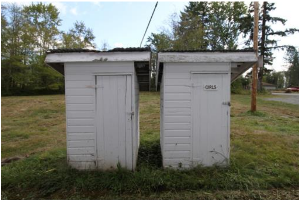
5 of 14. Front (west) elevation facing east of circa 1930s-era outhouses. Photo labeled as WA_SkagitCounty_HoogdalSchool_5.
