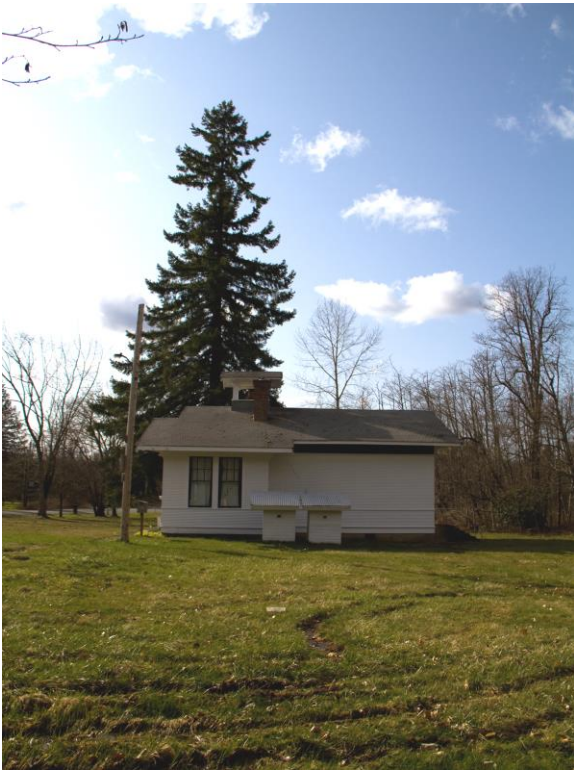
2 of 14. Side (east) elevation facing west 1916 schoolhouse and two WPA-era outhouses. Photo labeled as WA_SkagitCounty_HoogdalSchool_2.
