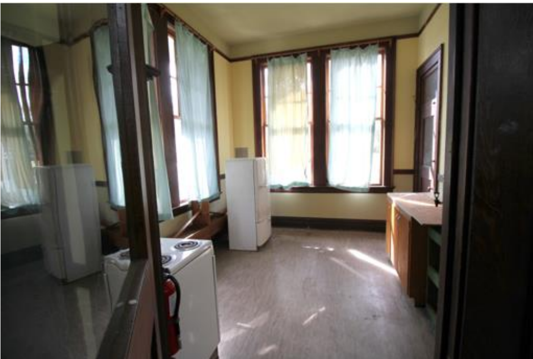
11 of 14. Interior of the teacher's office facing south. Photo labeled as WA_SkagitCounty_HoogdalSchool_11.
