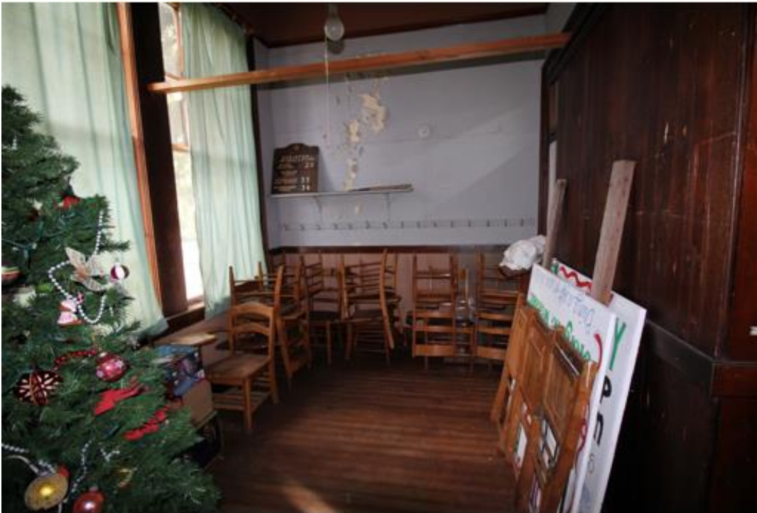
14 of 14. Interior of the cloakroom facing west. Photo labeled as WA_SkagitCounty_HoogdalSchool_14.
