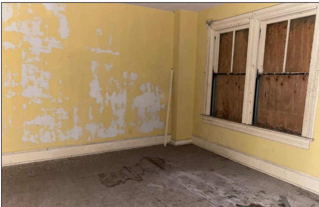
Photo 38 of 46: Keepers' Quarters south unit bedroom showing retained flooring, plaster, and partial window sash.
