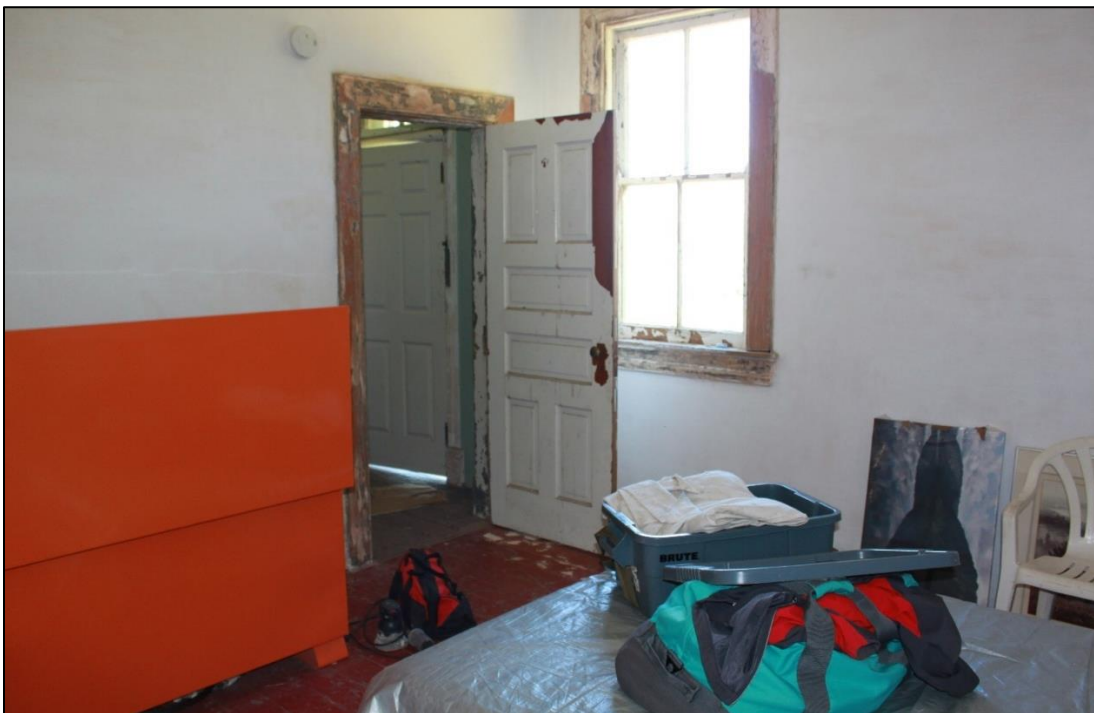
Photo 32 of 46: Keepers' Quarters north unit wood storage area (rear wing extension) showing original wood floors, windows, doors, and plaster work all retained.
