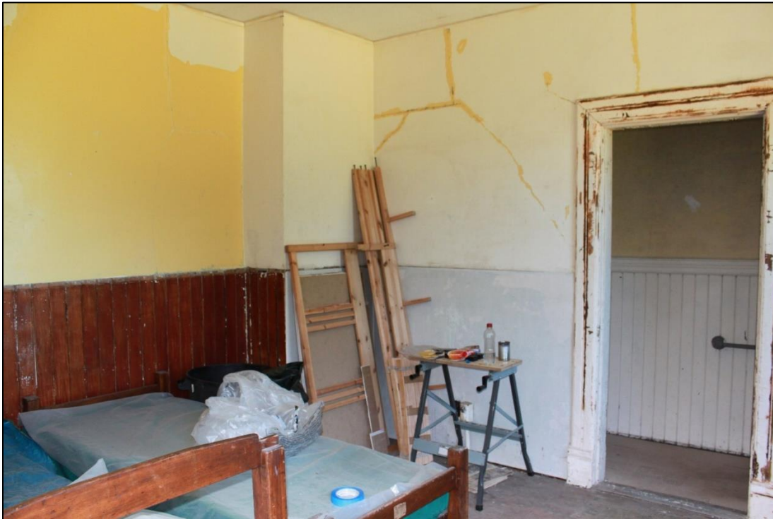
Photo 31 of 46: Keepers' Quarters north unit entry hall showing in-progress restoration work and retained plaster, flooring, and door surround.
