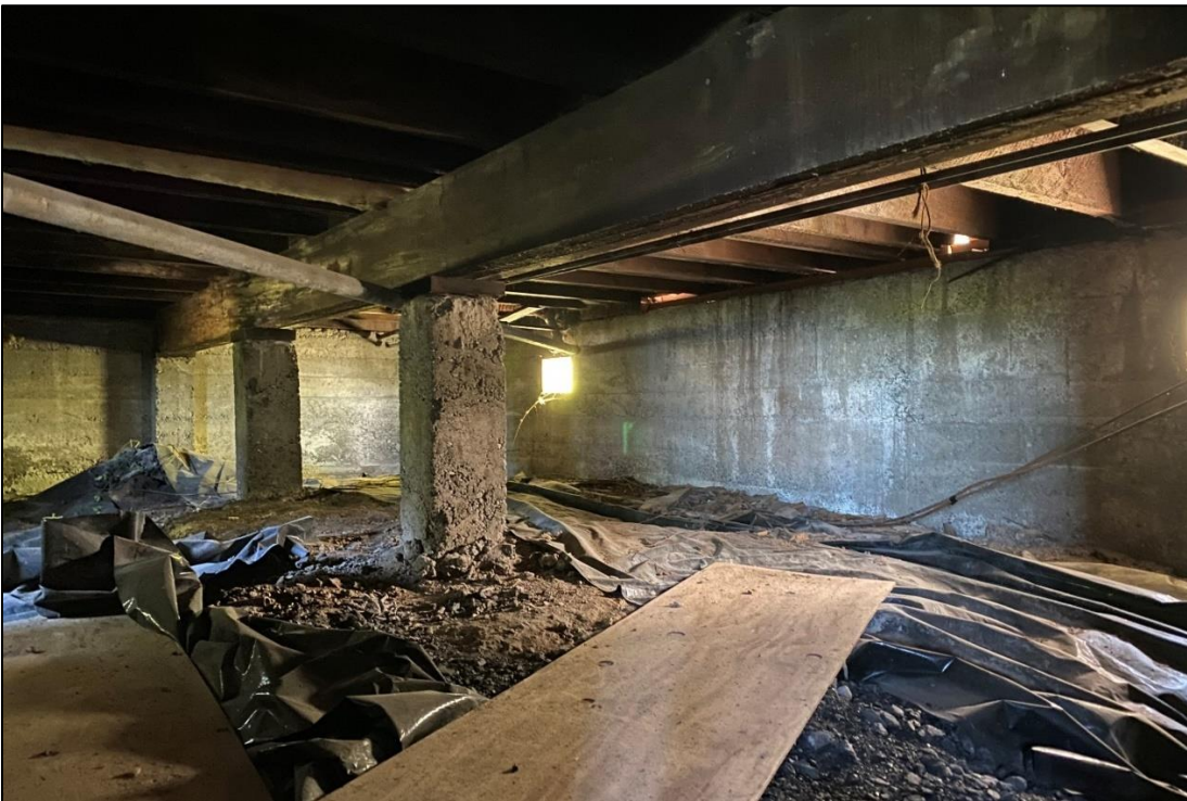
Photo 26 of 46: Keepers' Quarters crawl space under north unit showing square concrete posts that support the rear wing extensions.
