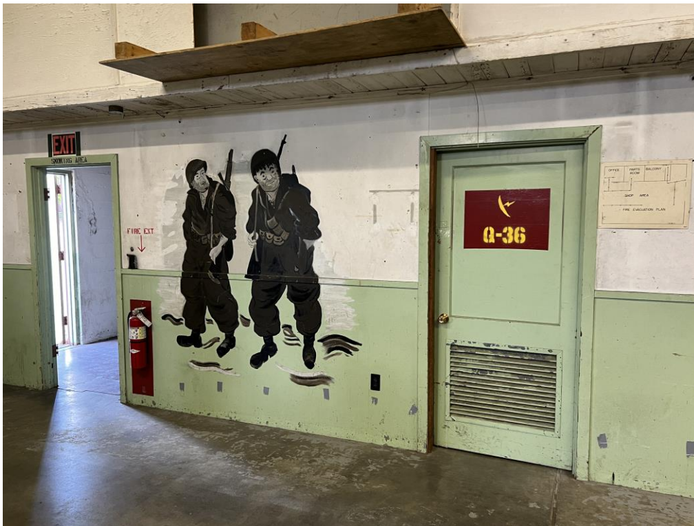
20 of 22 (WA_Thurston_NationalGuardArmoryOlympia_0011) Interior view detail of the Vehicle Storage Building showing "Willie & Joe" artwork.
