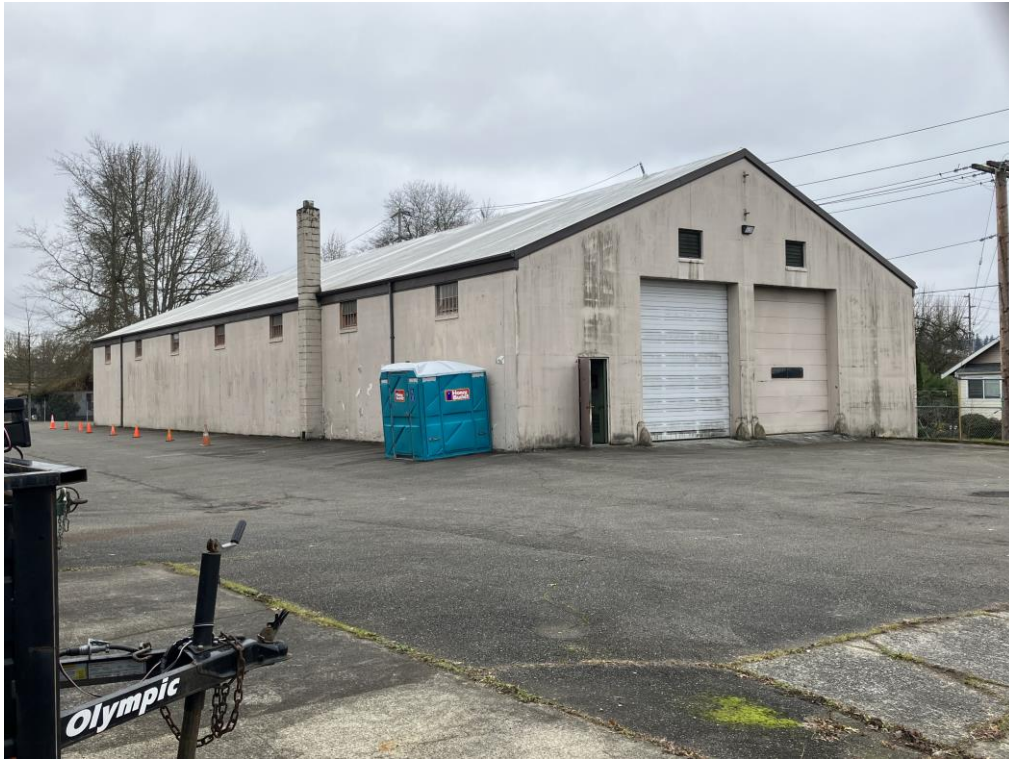
18 of 22 (WA_Thurston_NationalGuardArmoryOlympia_0011) View of the Vehicle Storage Building looking southeast.
