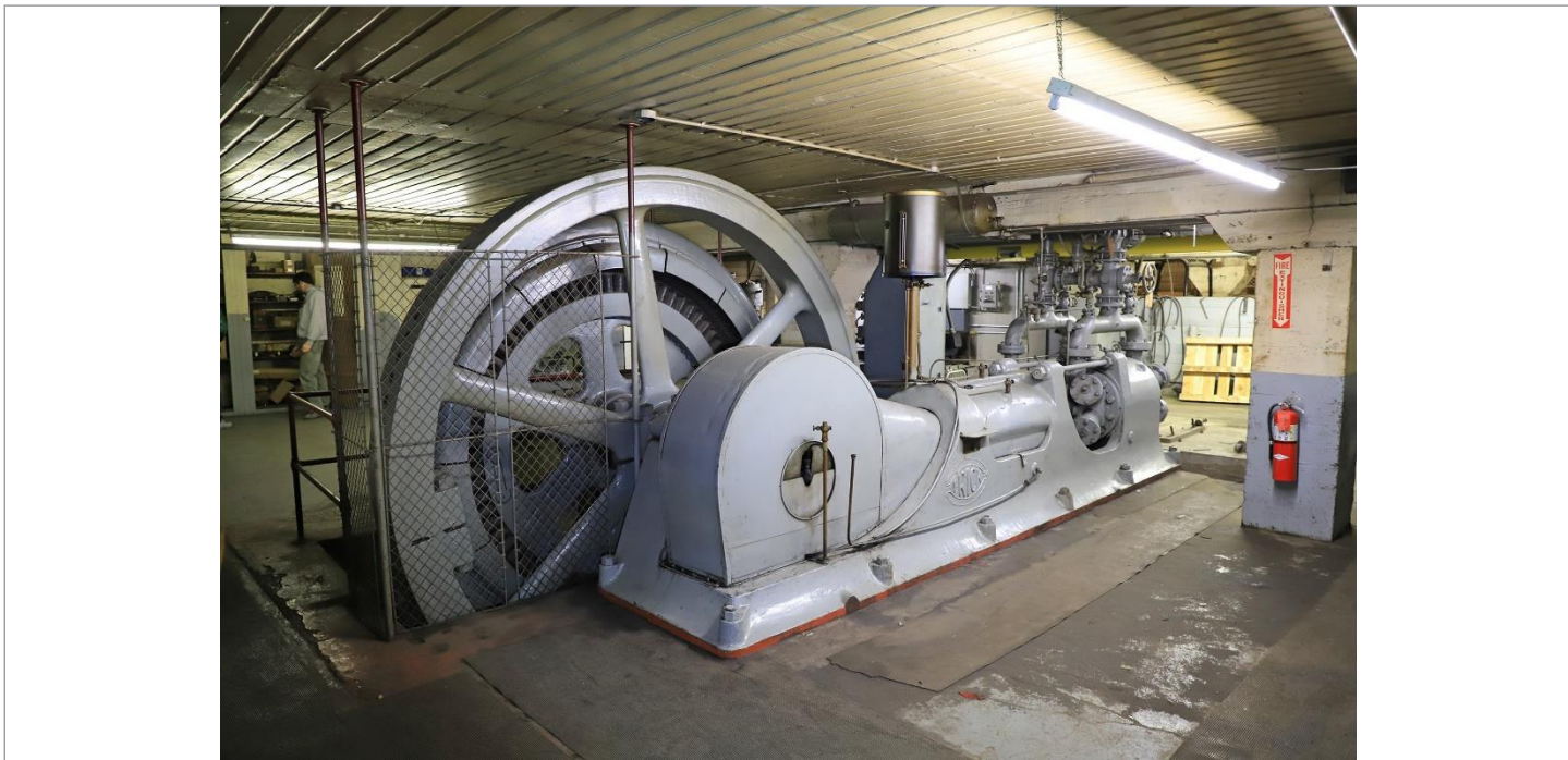
WA_Yakima County_Fruit and Produce Row_0025. Ammonia compressor in basement of 201 N First Avenue.
