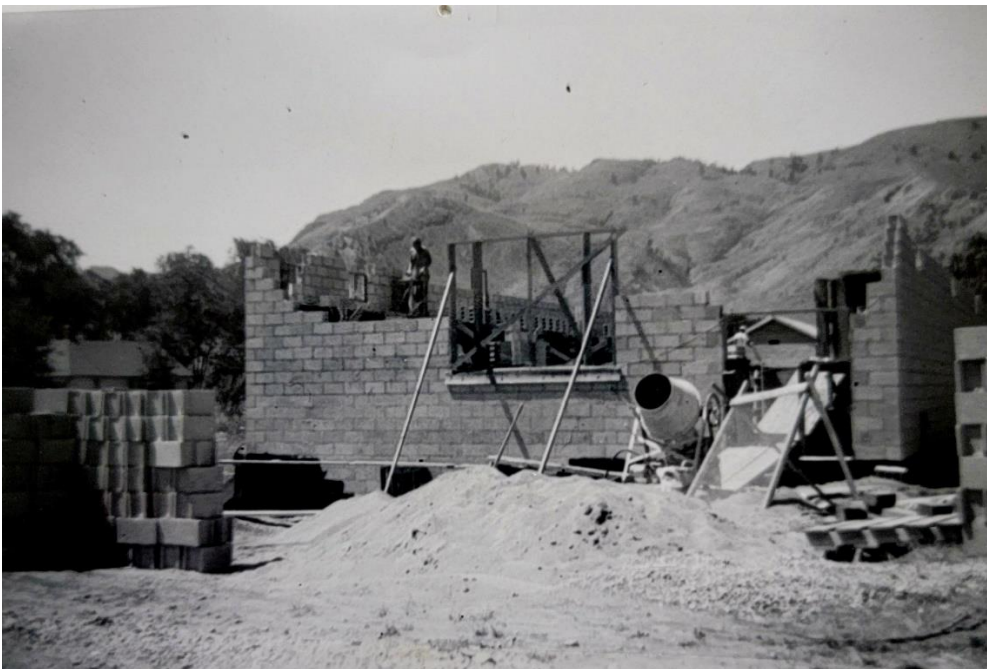
Grange Archives, Façade Wall Construction, 1957.
