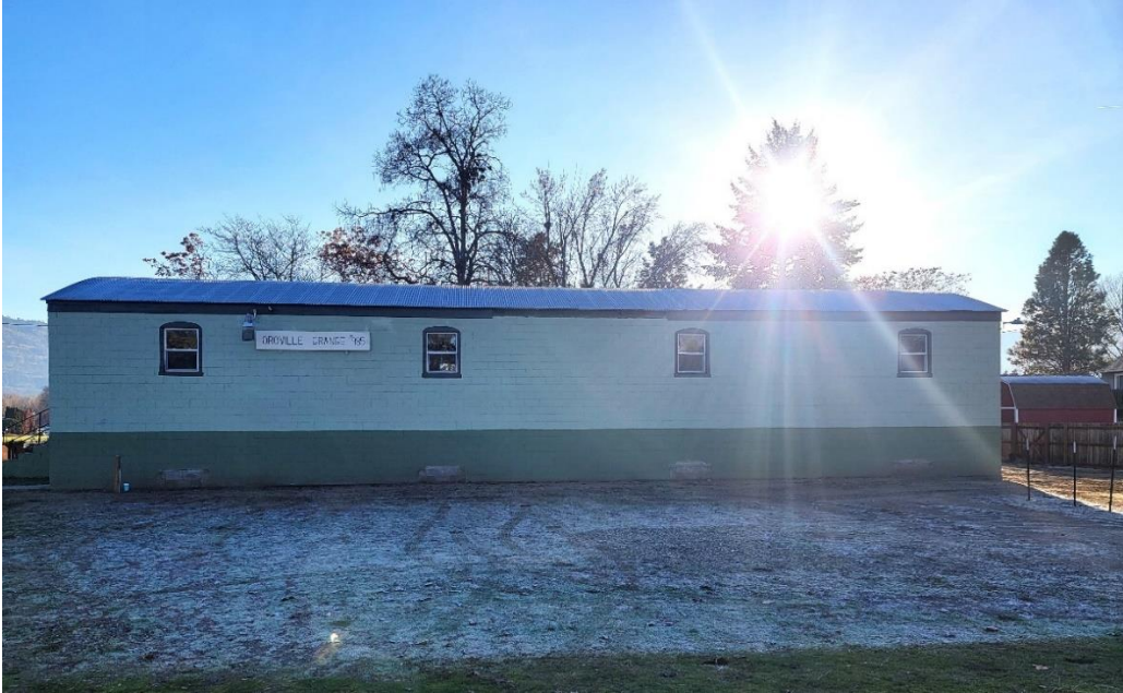
North Elevation looking south.
