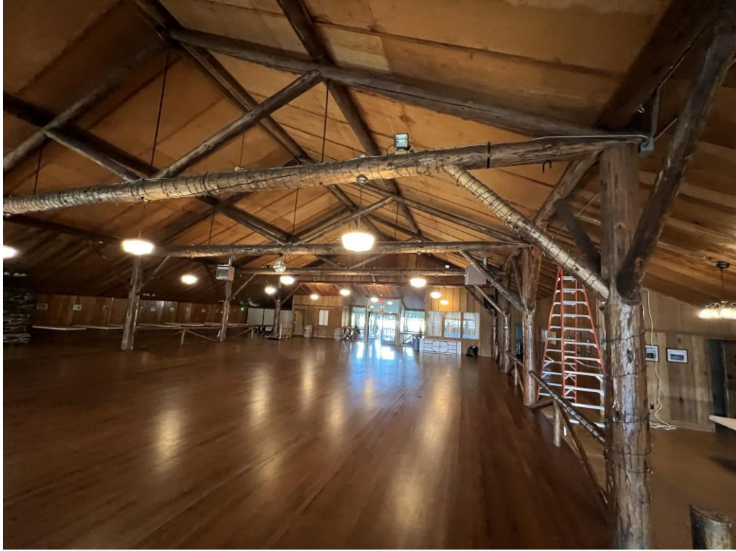
Dance hall view to the north towards main entry.
