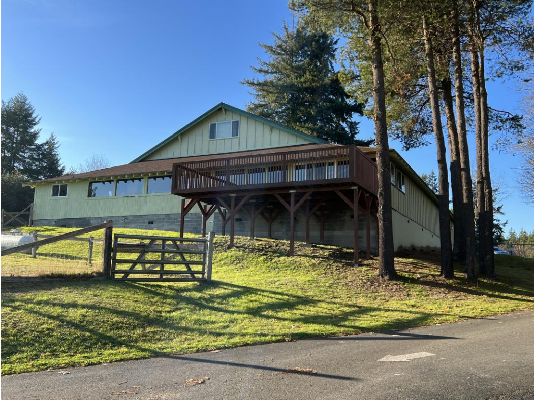
Rear / Southeast facade.
