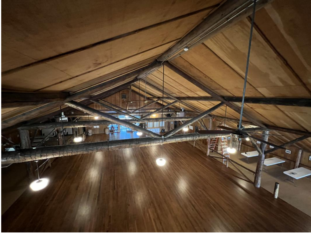
Detail of open truss system.
