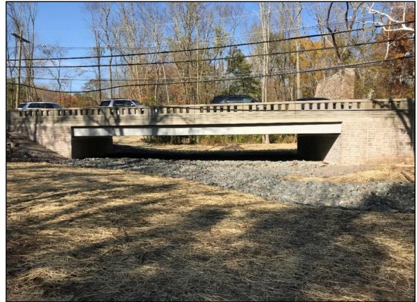
*A three-span concrete-encased steel stringer bridge (left) was replaced with a single-span concrete slab beam bridge (right). (Images Courtesy of Urban Engineers).*
