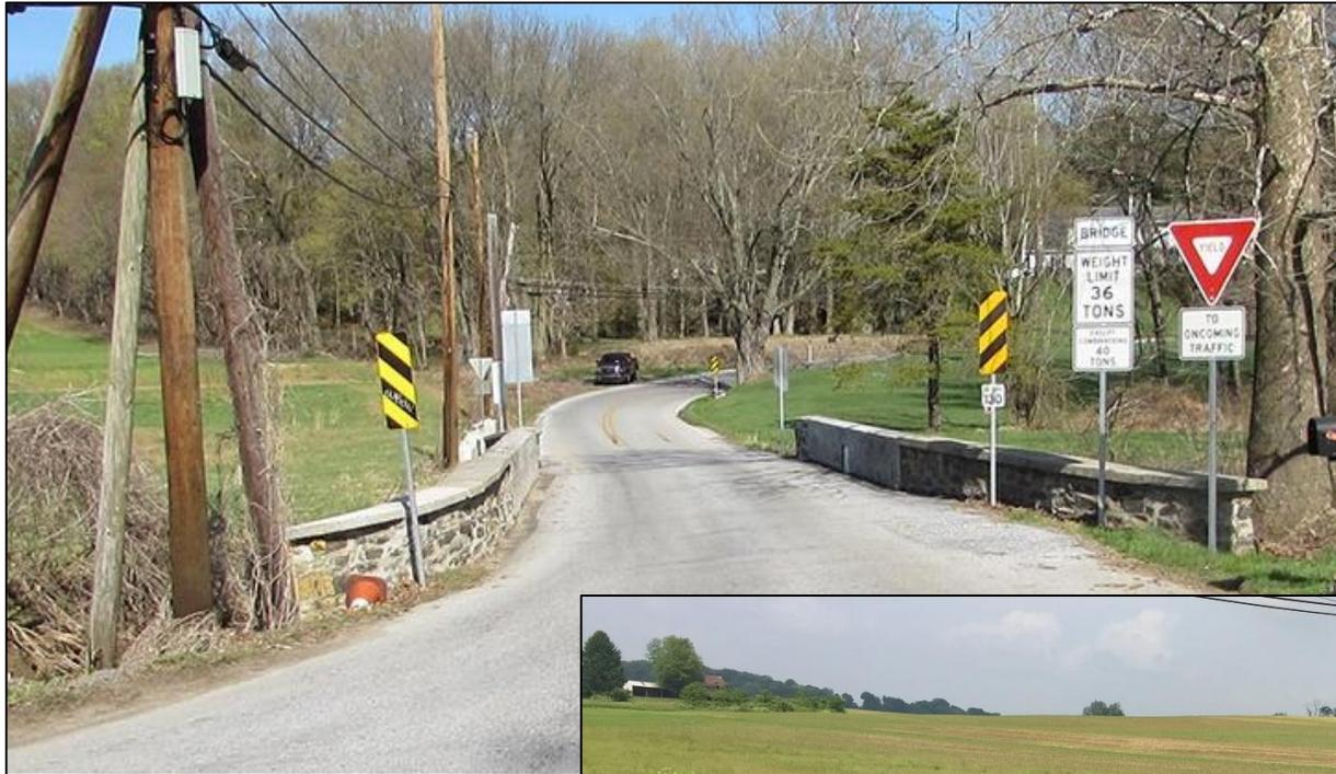
*As part of the Pennsylvania Rapid Bridge Replacement Program, the standard replacement design can be enhanced with the use of form liners (below) to achieve compatibility when the existing bridge (left) is set within a historic district.*
