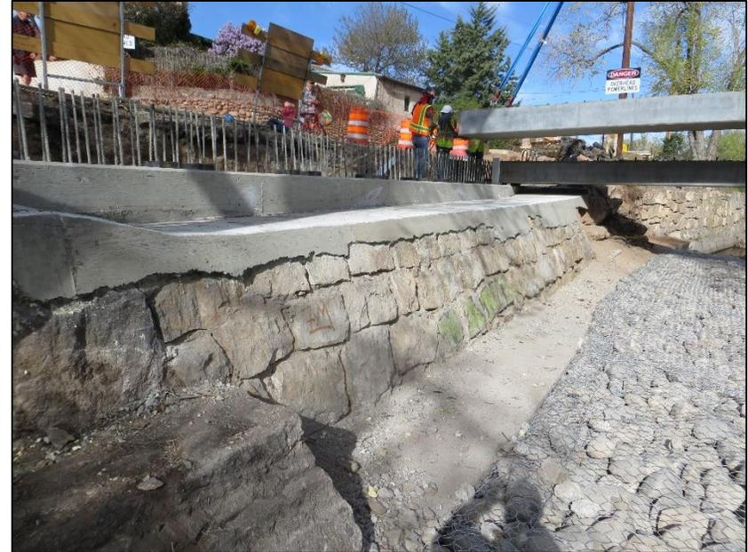
*A two-span, concrete channel beam bridge with rock masonry abutments and pier (left) replaced with a single-span concrete bridge, retaining the original stone abutments (right). A concrete sill was applied to the tops of the existing abutments to create a level surface for the new beams. (Images: courtesy of WSP).*
