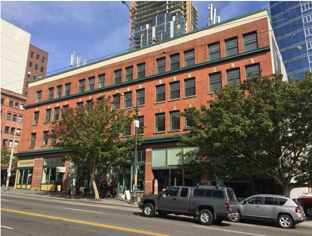
2 of 16. Colonnade Hotel 107 Pine Street, Seattle, King County, WA Photo: The Johnson Partnership, October 5, 2016. Western façade.
