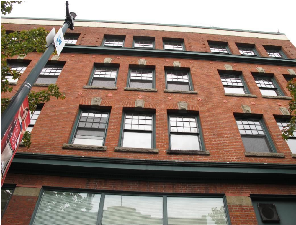
8 of 16. Colonnade Hotel 107 Pine Street, Seattle, King County, WA Photo: The Johnson Partnership, October 5, 2016. Detail at northern façade.
