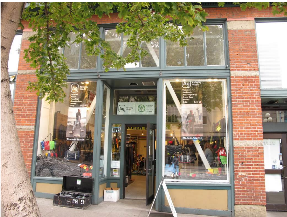
9 of 16. Colonnade Hotel 107 Pine Street, Seattle, King County, WA Photo: The Johnson Partnership, October 5, 2016. Detail at storefront.
