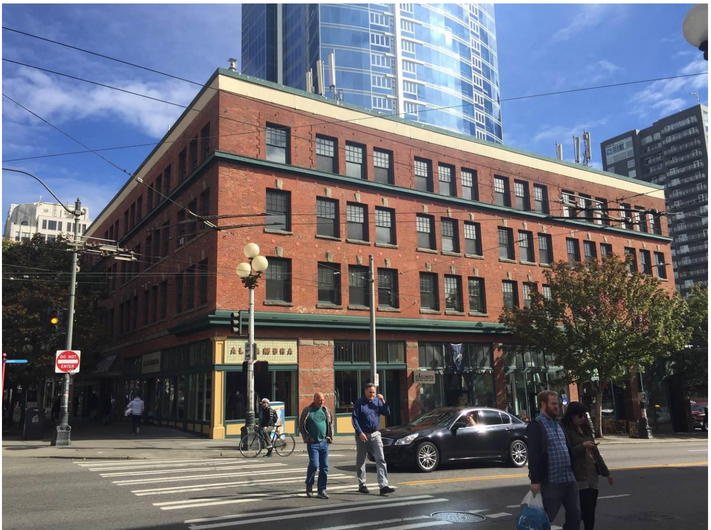
1 of 16. Colonnade Hotel 107 Pine Street, Seattle, King County, WA Photo: The Johnson Partnership, October 5, 2016. Western façade.
